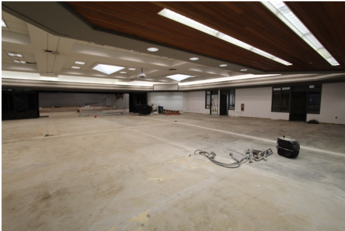
South Lake MS: Modernization
