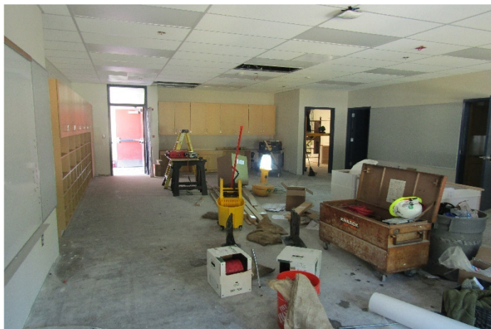
Plaza Vista School: Renovations
