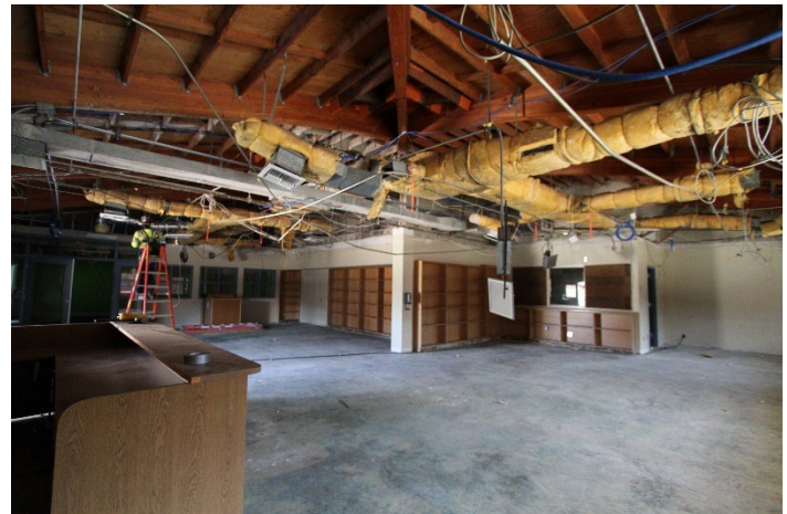
University Park ES: Renovation
