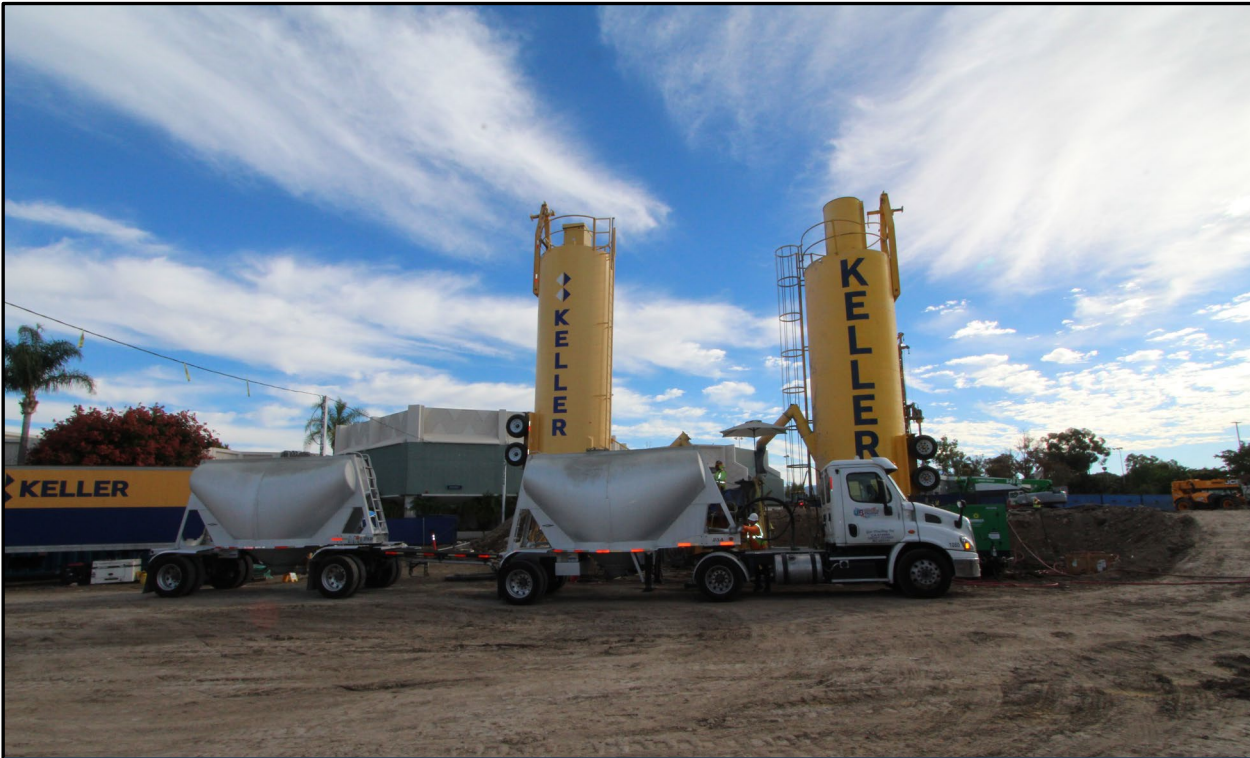
Increment No. 1: Ground improvements
