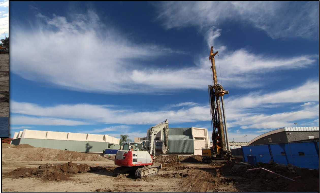
Increment No. 1: Ground improvements
