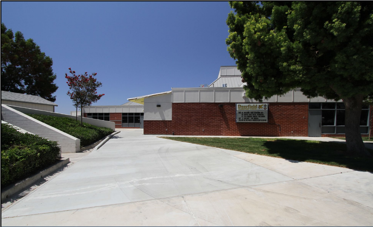
Expansion and site improvements
