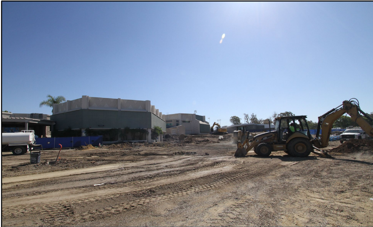
Relocation and installation of underground utilities
