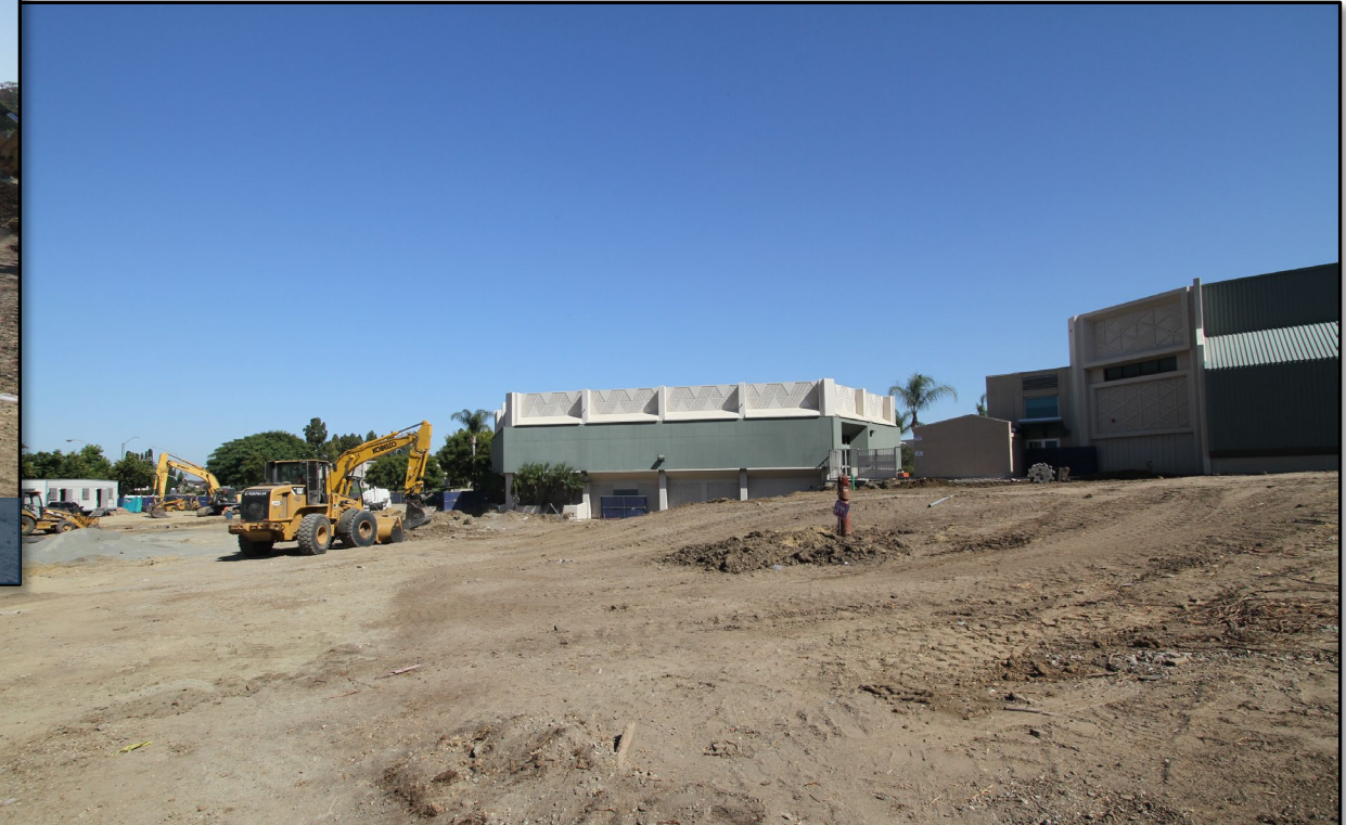
Relocation and installation of underground utilities
