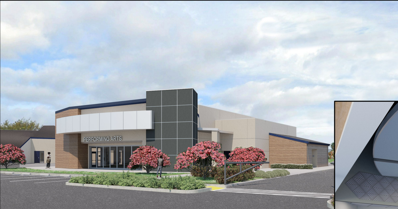
Exterior of new Multipurpose Building
