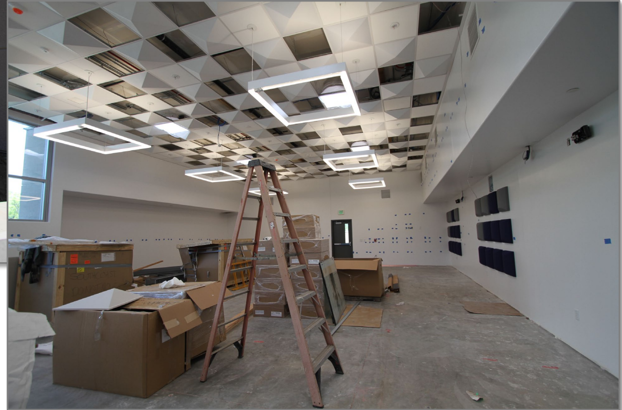
Music classroom expansion (interior)
