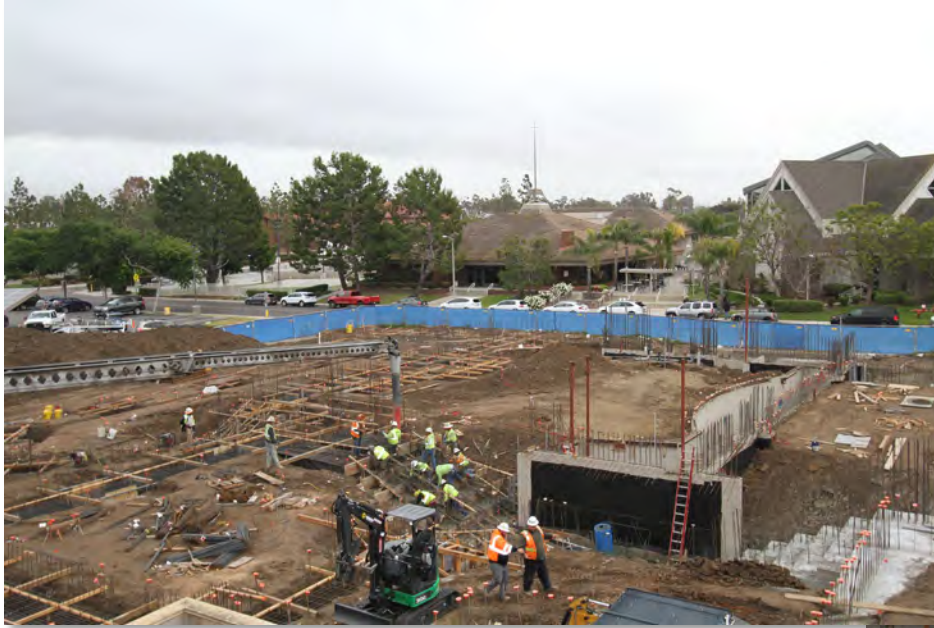
Concrete placement for footings
