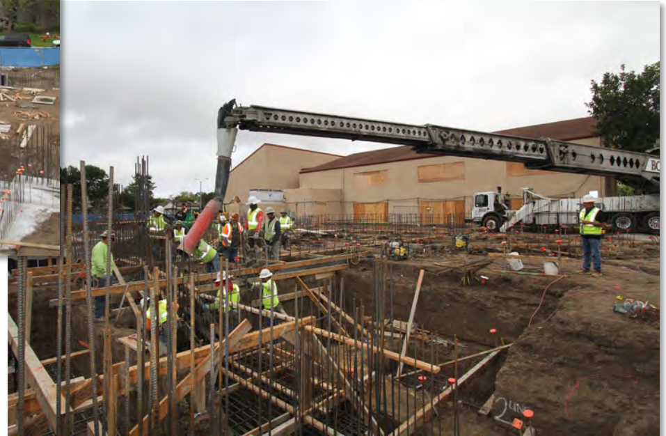
Concrete placement for footings
