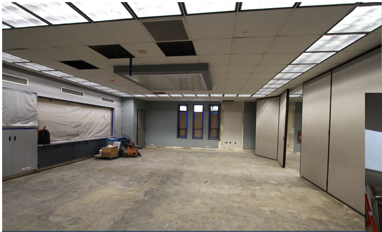
Interior of Modernized Classroom
