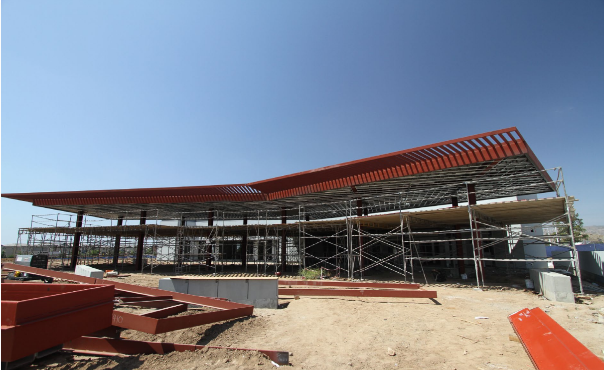
Exterior of Nutrition Services/ICCP (Building D)
