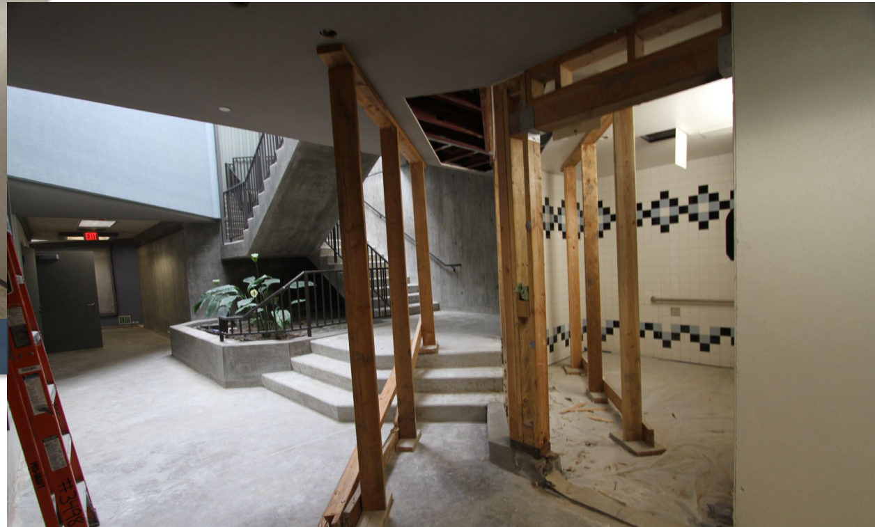
Interior of Restroom Improvements
