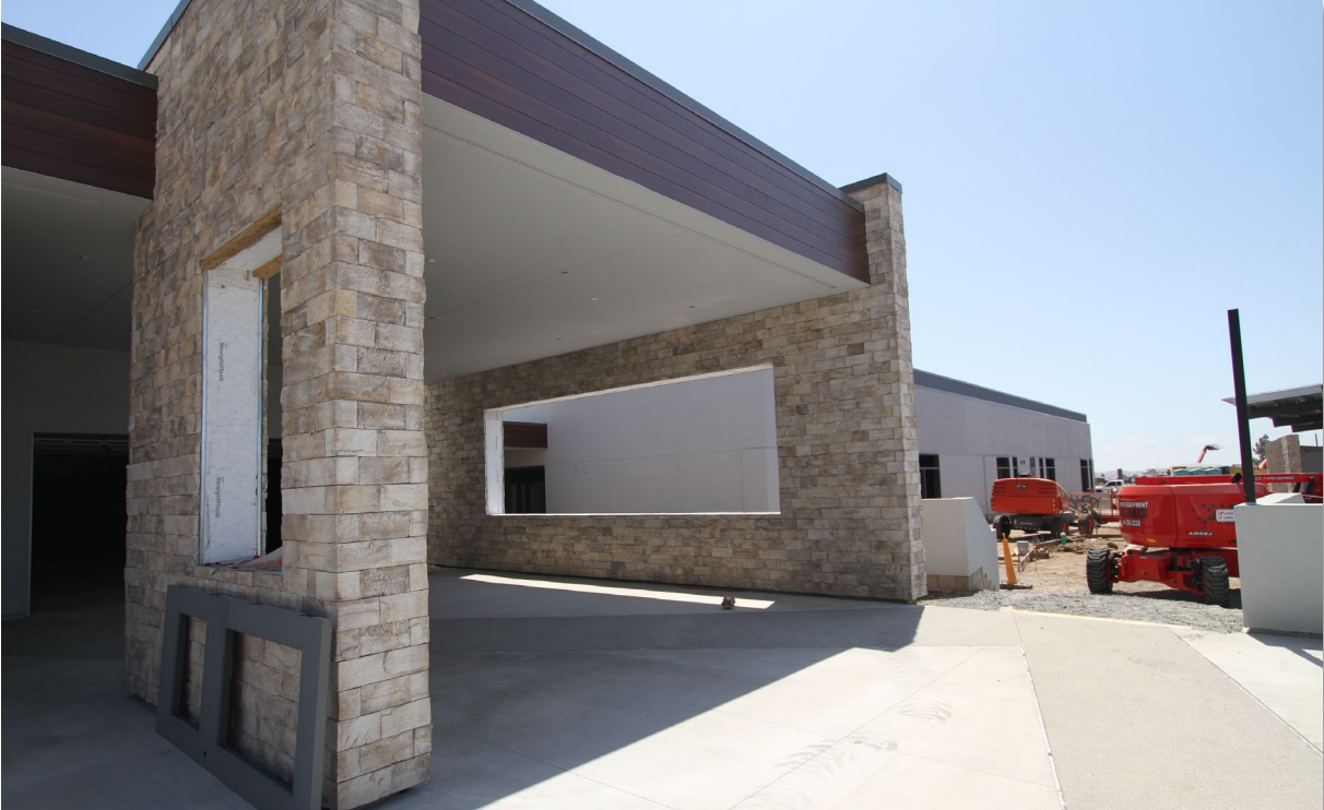
Kindergarten Lunch Area (Building A)
