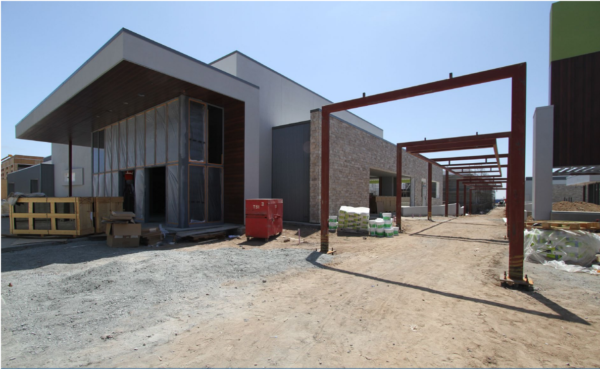
Exterior of Multipurpose/Music (Building B)/Walkway
