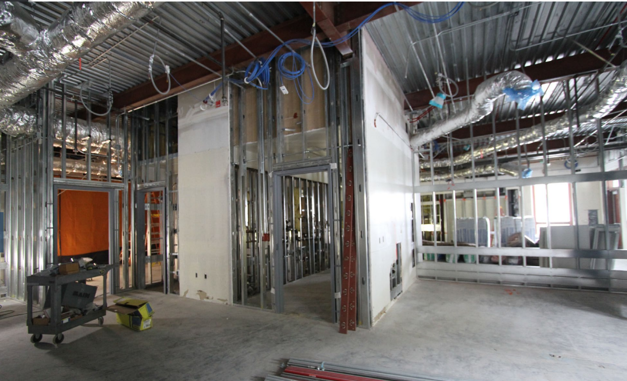
Interior of Kindergarten Classrooms
