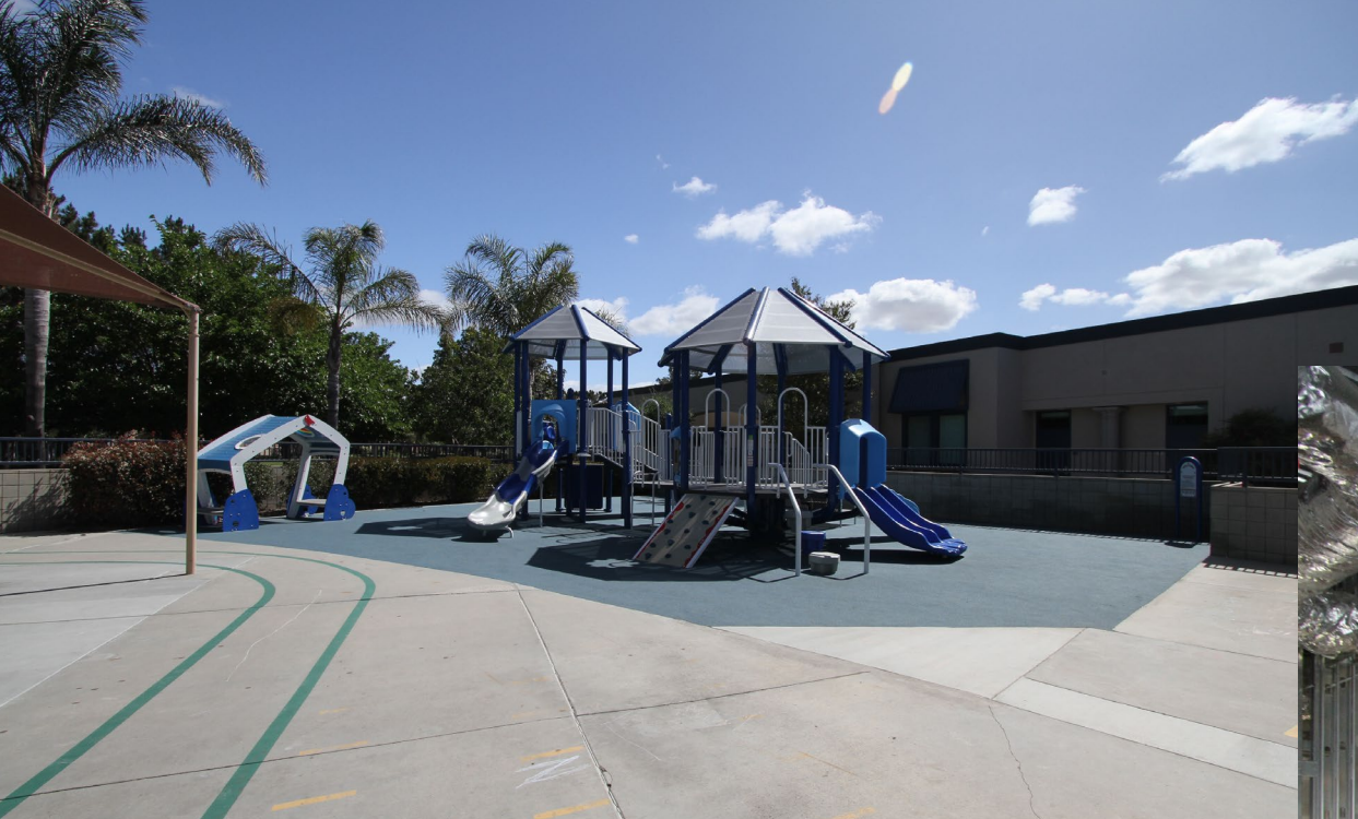
New Kindergarten Play Equipment
