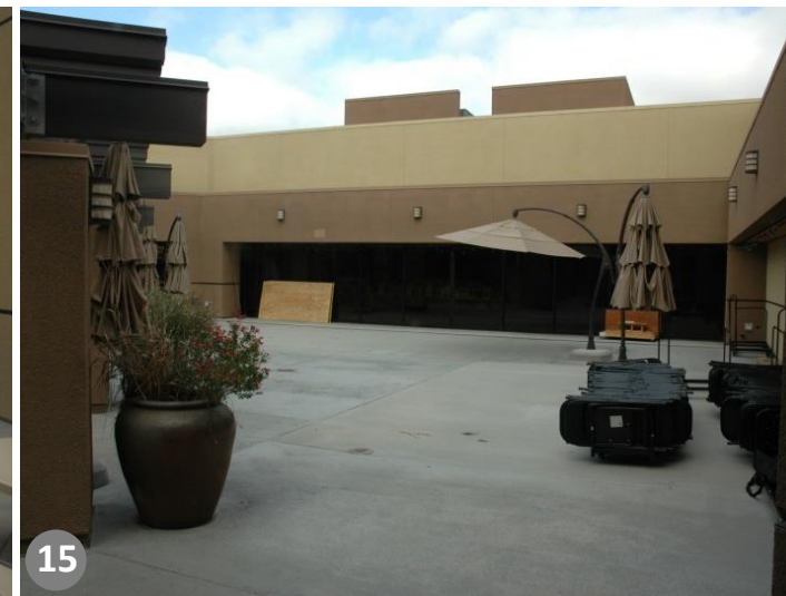
Central Courtyard near MPR
