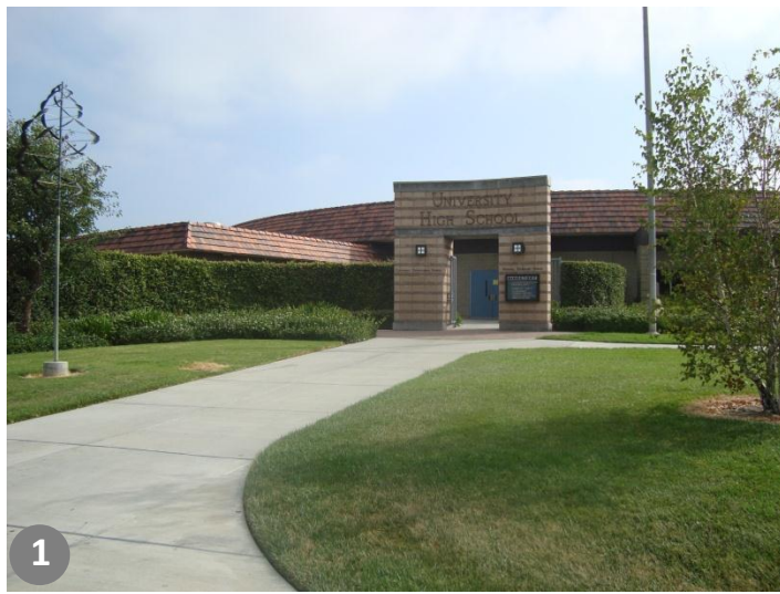
Entrance to Admin. Building (near DHH offices)
