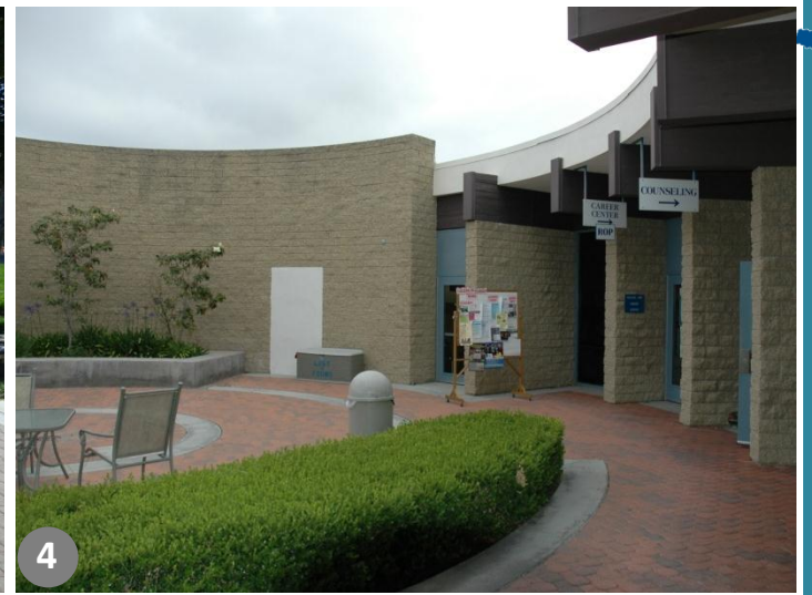
Central Courtyard, Admin. Building
