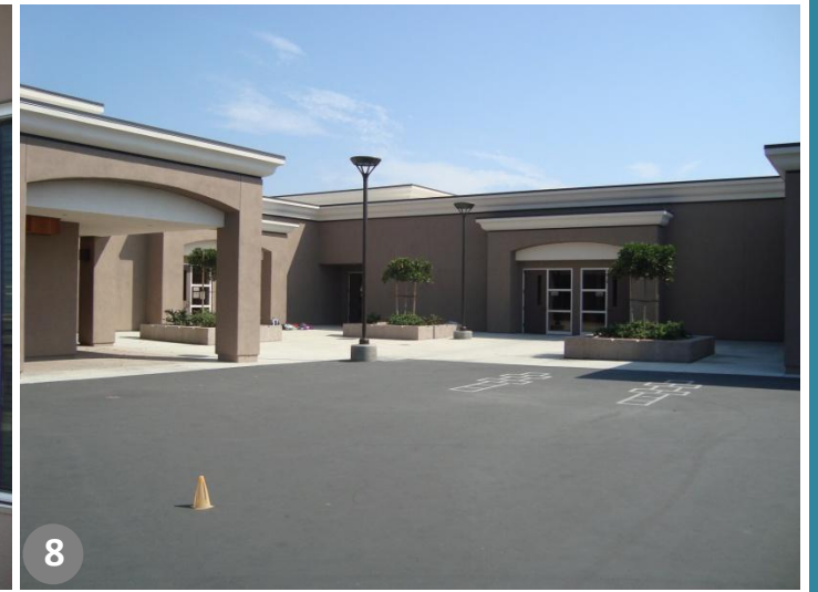
8 Classroom Courtyard Area
