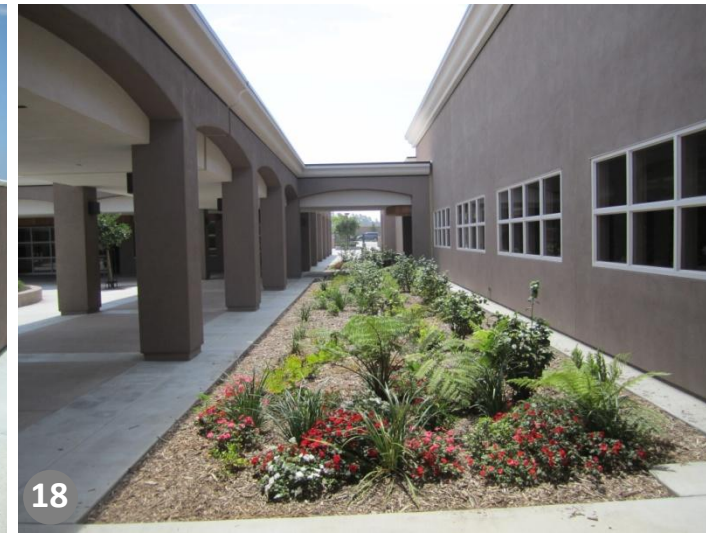
Central walkway and landscaping
