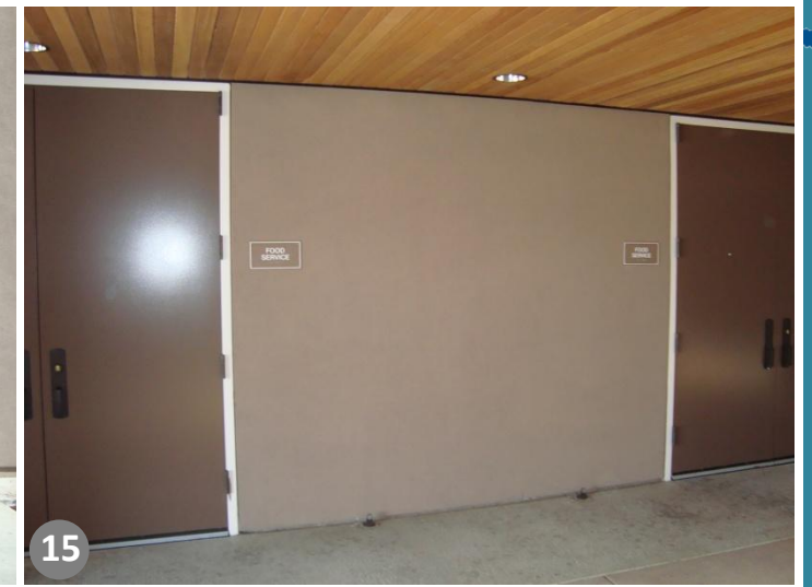
Outdoor access/entry to Food Service
