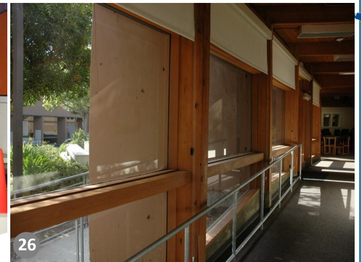
Hallway in Classroom Wing
