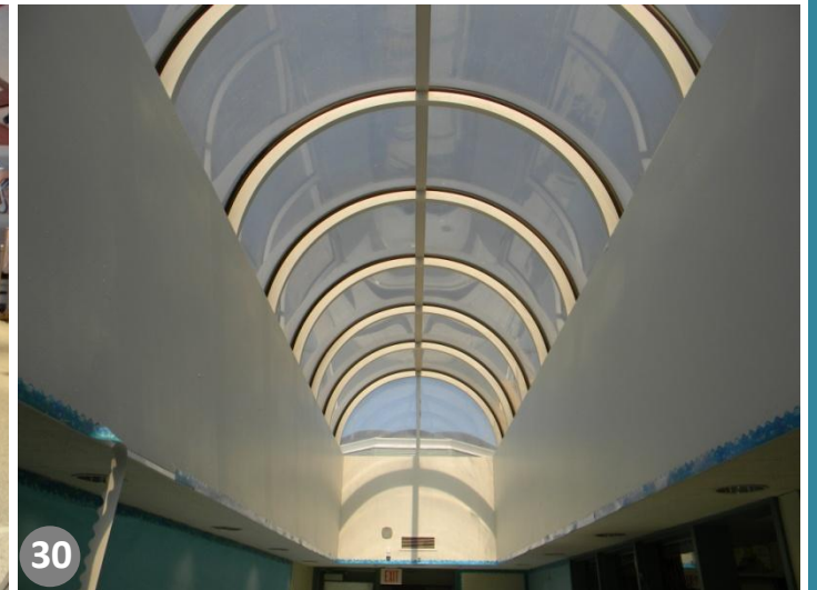
Skylight in each Pod
