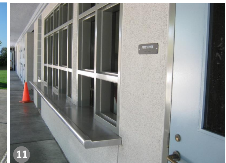
Exterior Food Service windows
