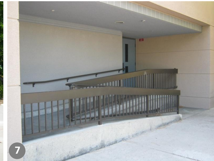
Ramp to MPR backstage area
