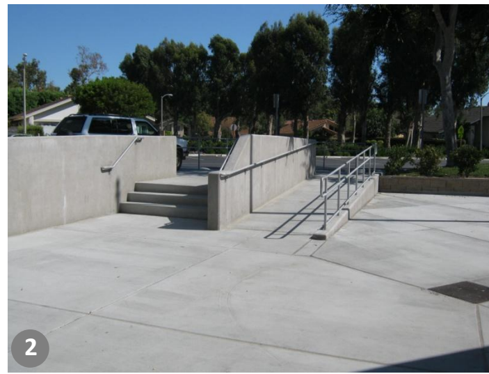
Front Ramp and Steps from Parking Lot
