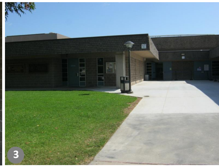
3 Entry to Administration and MPR
