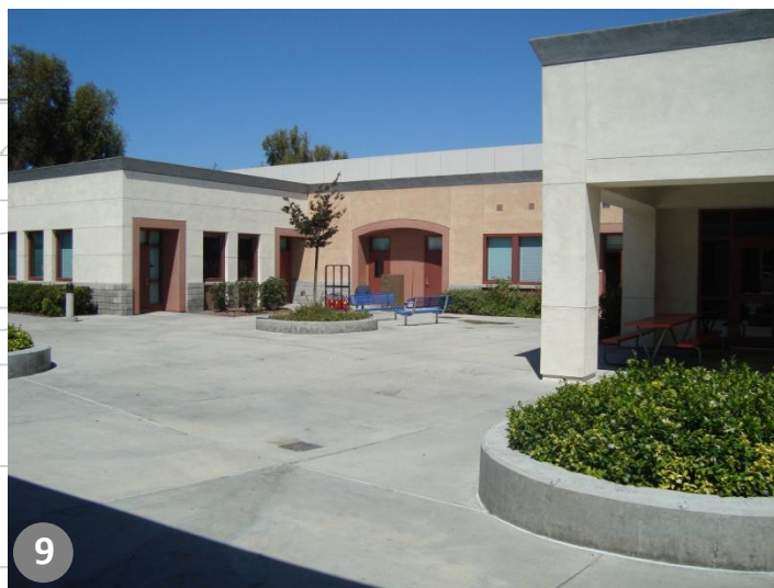
Typical classroom courtyard
