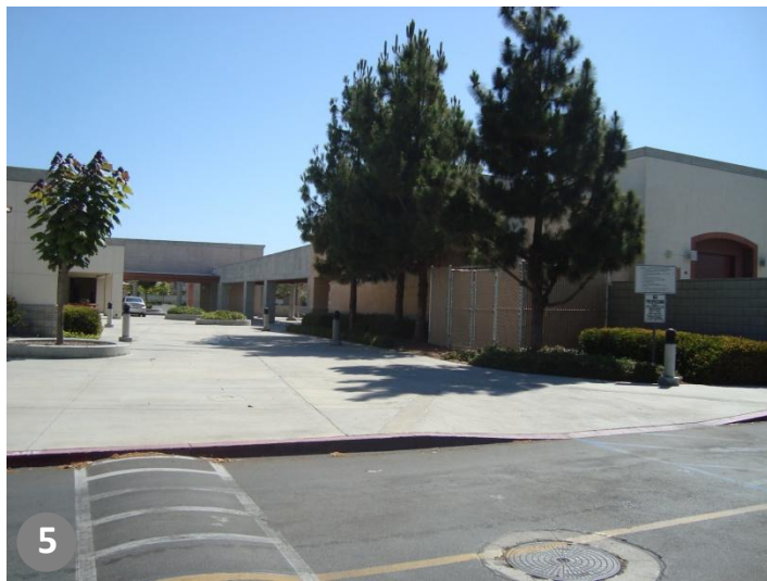
Walkway between MPR and main building
