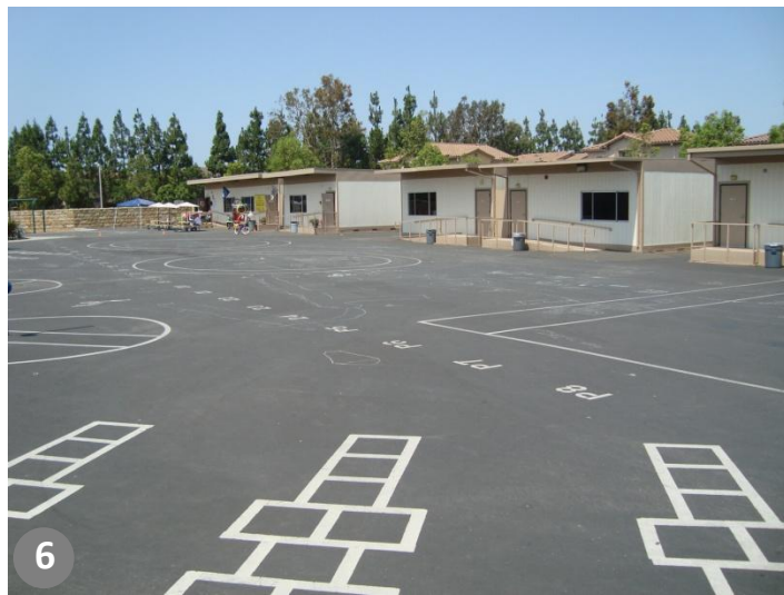
Classroom Portables and Childcare Portables on western side of site
