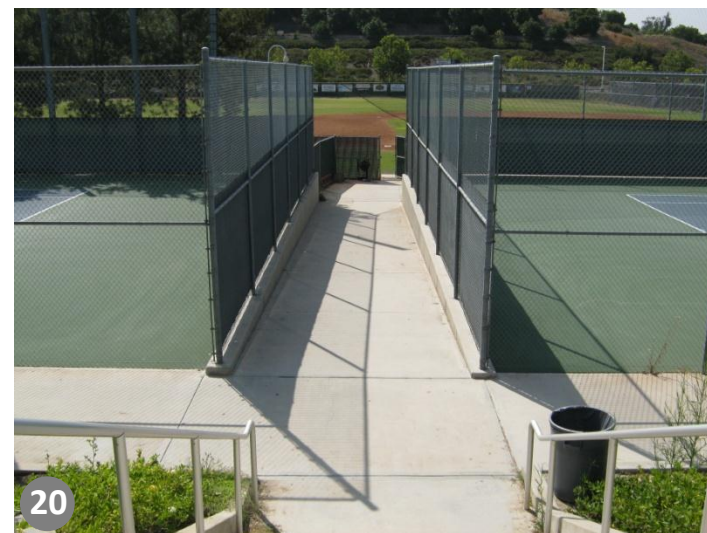
20 Access to Tennis Courts
