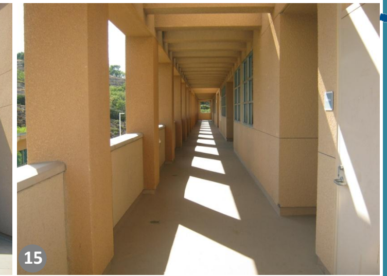
15 Typical Exterior Hallway
