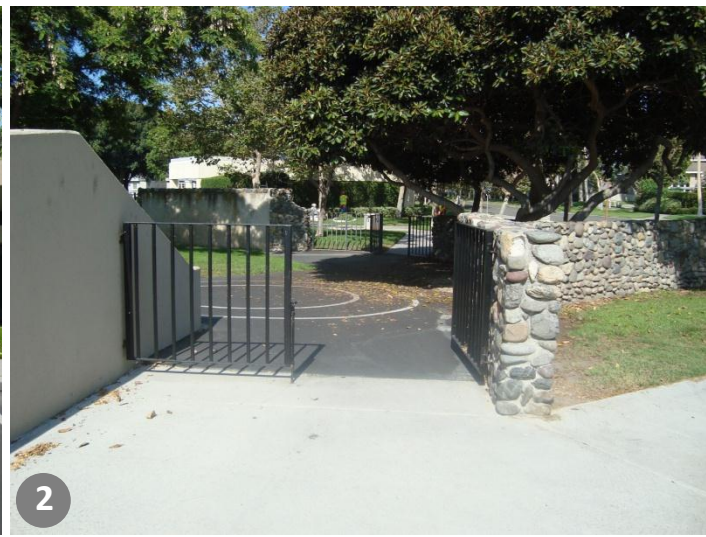
2 Entrance near Kindergarten Play Area
