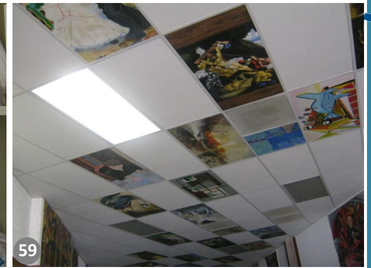
Ceiling in Unified Arts Hallway
