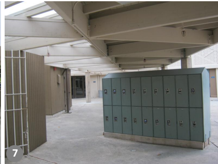
Covered Locker Area
