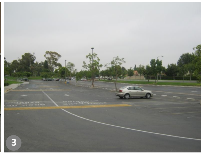
Main Parking Lot
