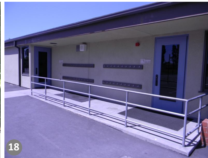
Covered Walkway between two Classrooms
