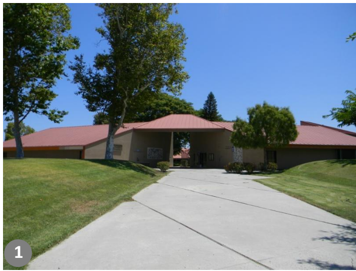
1 Front of School on Paseo Westpark
