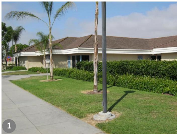
Sidewalk near Main Entry
