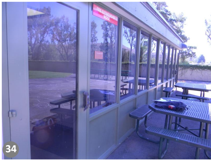
34 Windows along Kindergarten Classroom wall
