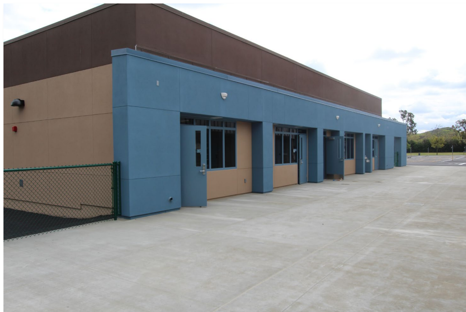
New science classroom building
