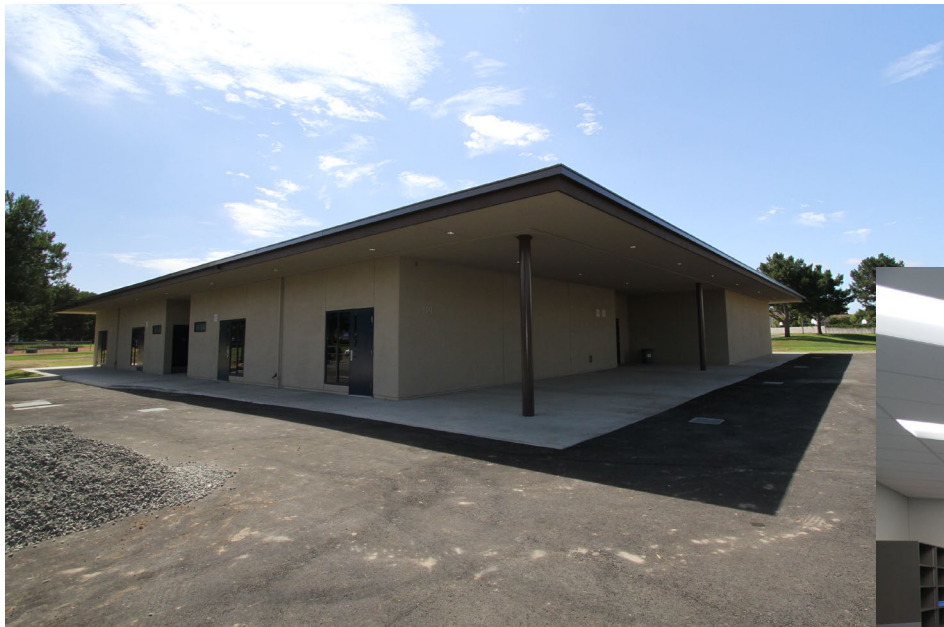
New science classroom building
