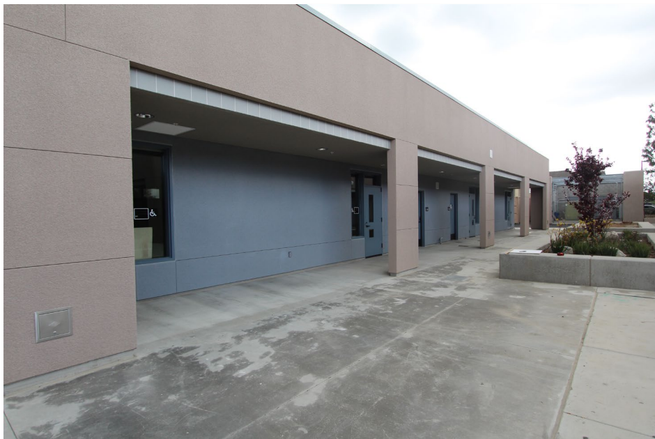
New science classroom building
