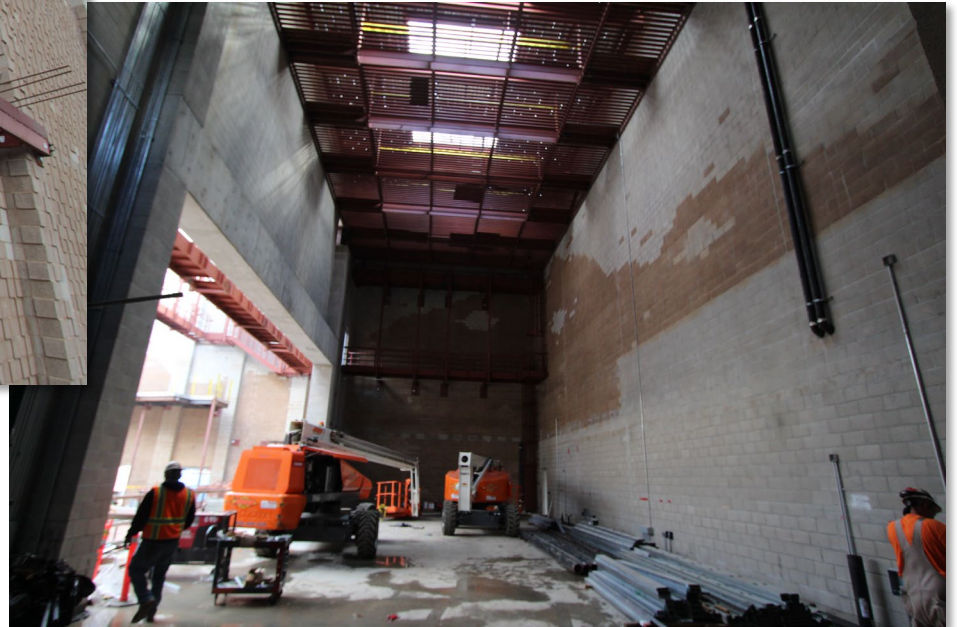
Interior view at back of stage (Fly Loft)
