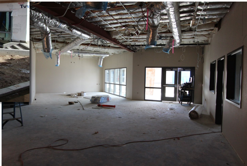
Interior view of expansion
