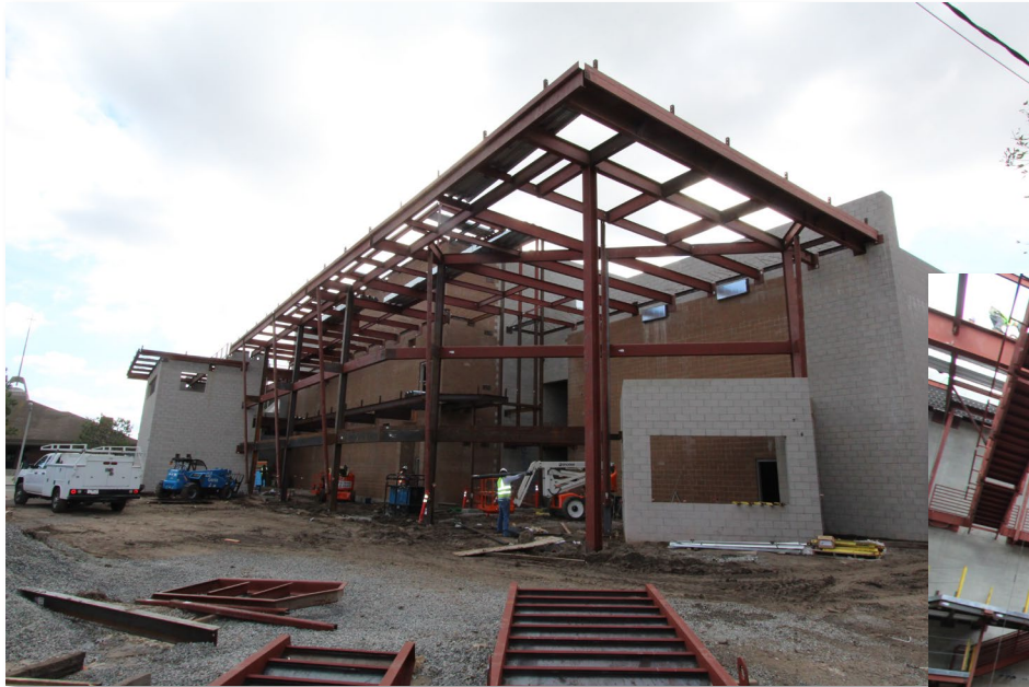
Building view from school
