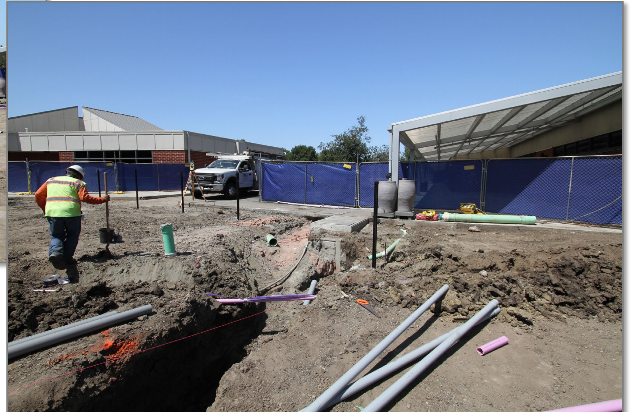
Underground utilities for new building
