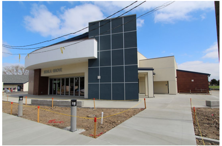
Culverdale ES: New Multipurpose Building
