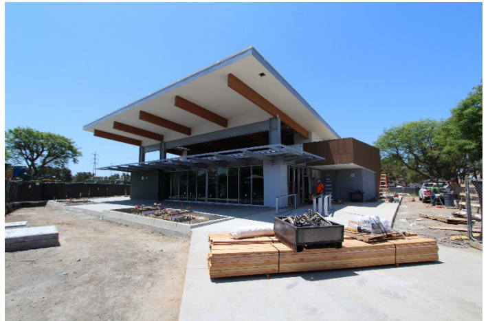
Greentree ES: New Multipurpose Building
