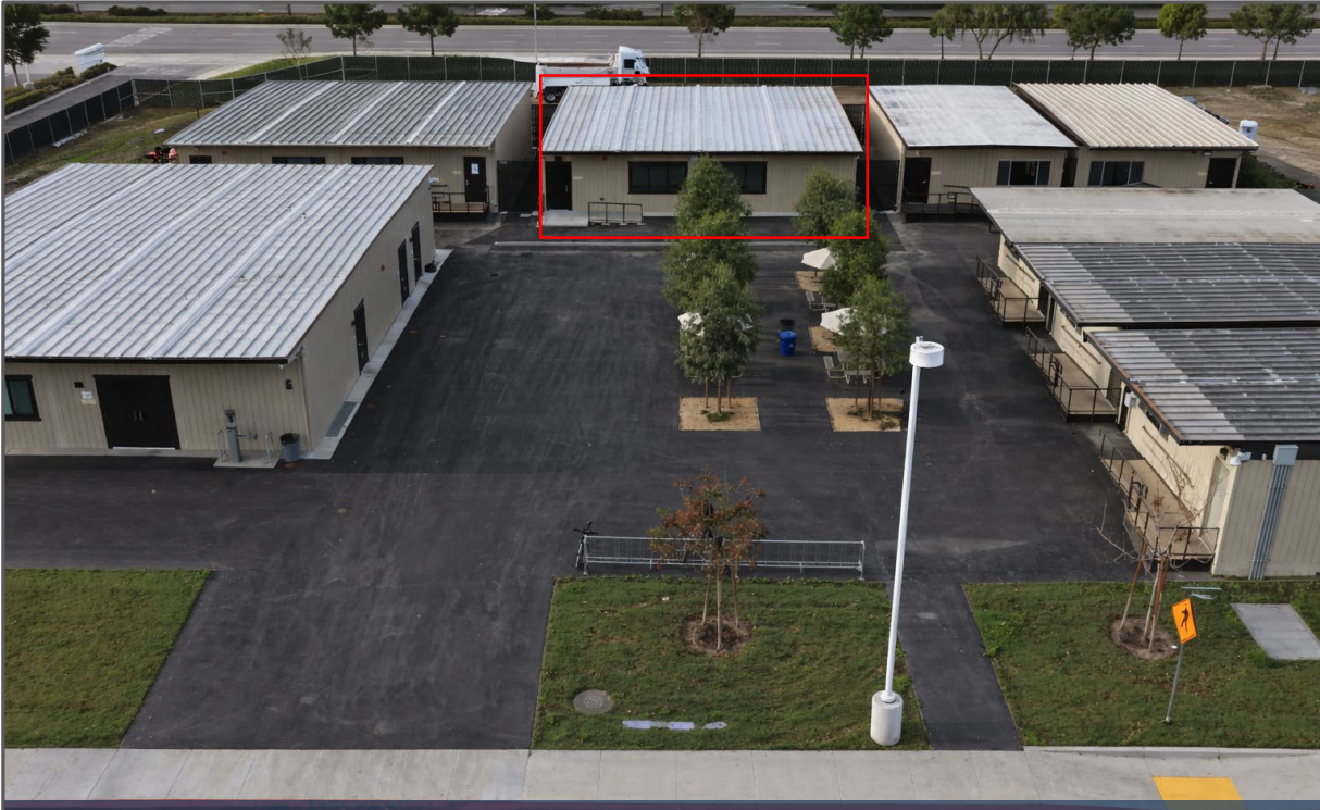
Aerial – Information Technology Building
