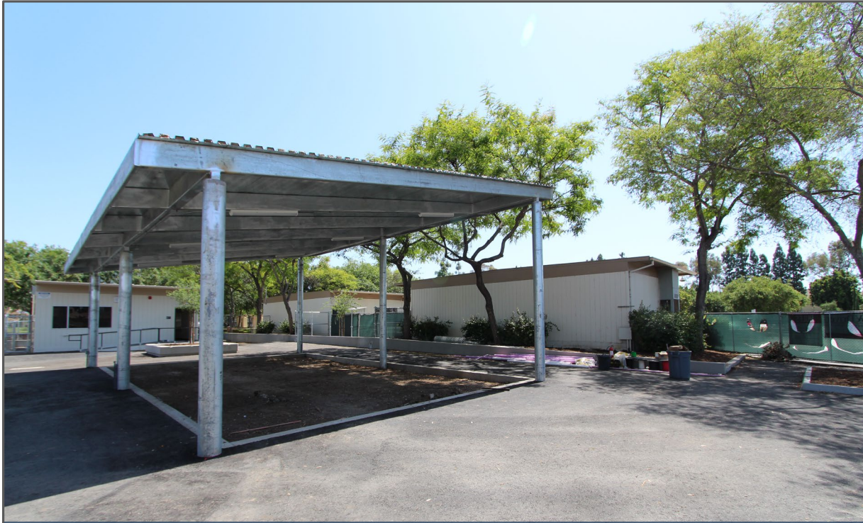
Exterior – New Lunch Shelter with Solar Array
