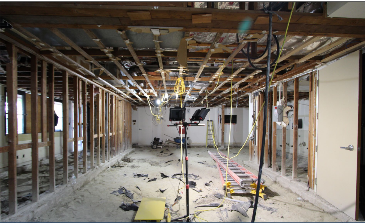
Nutrition Services – Demolition of Speedline Area
