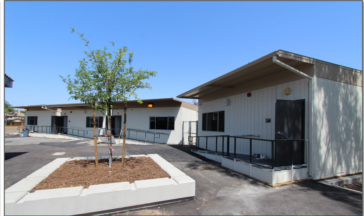
Exterior – Relocated Relocatable Classrooms (4 Relos)
