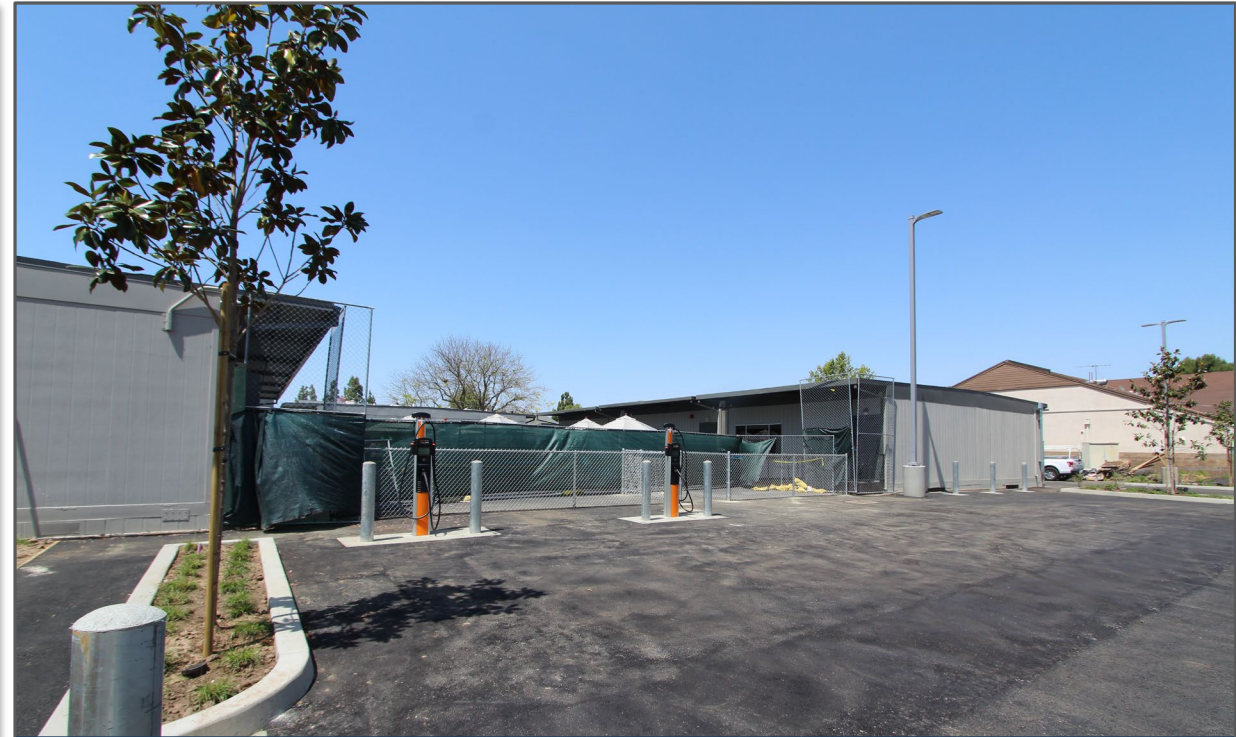
Exterior – Expanded Parking Lot with EV Charging Stations
