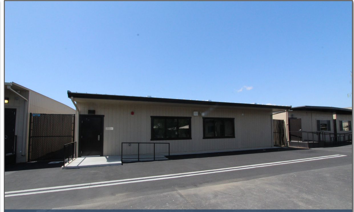
Exterior – Information Technology Building
