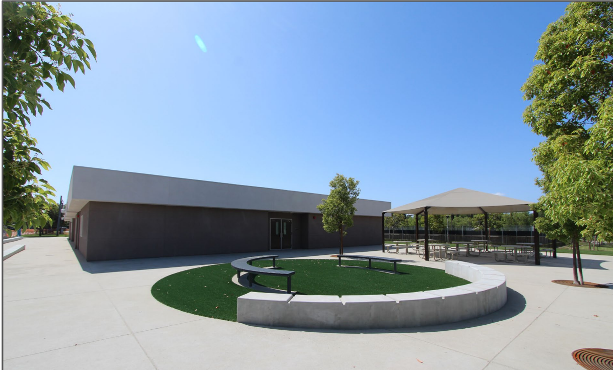
Exterior – New Building and Outdoor Learning Area
