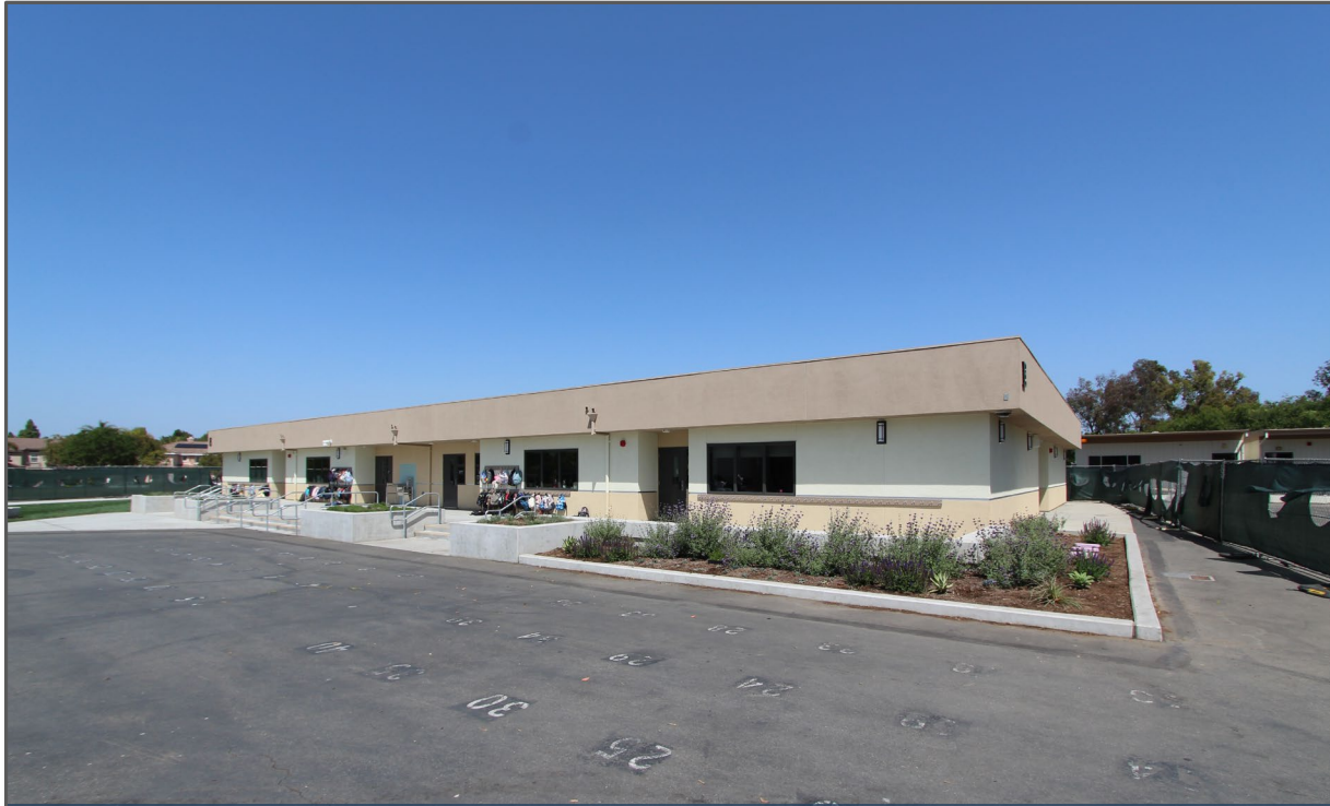
Exterior – New Classroom Building
