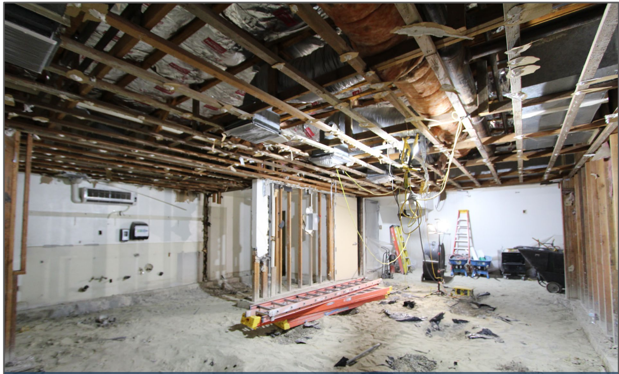
Nutrition Services – Demolition of Speedline Area
