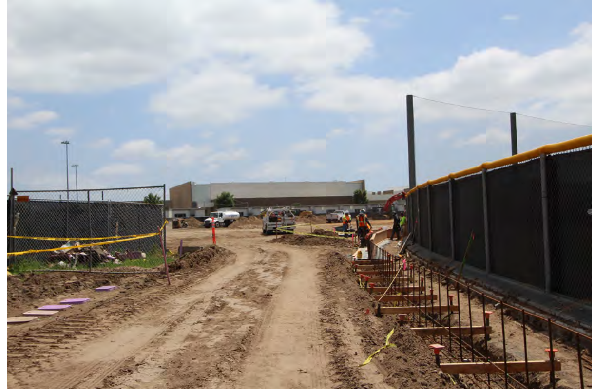
Portola HS Field Renovation – Formwork for curbs/low wall.
