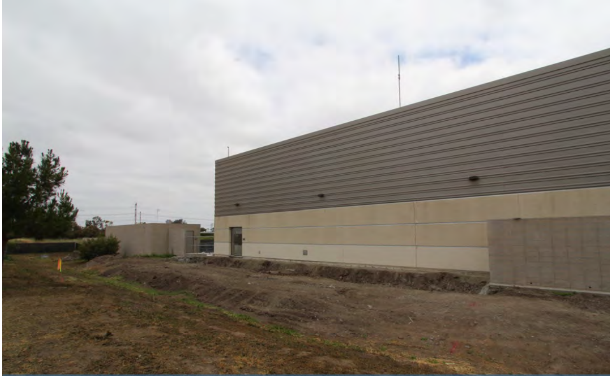
Nutrition Services – Freezer and Refrigeration Expansion
