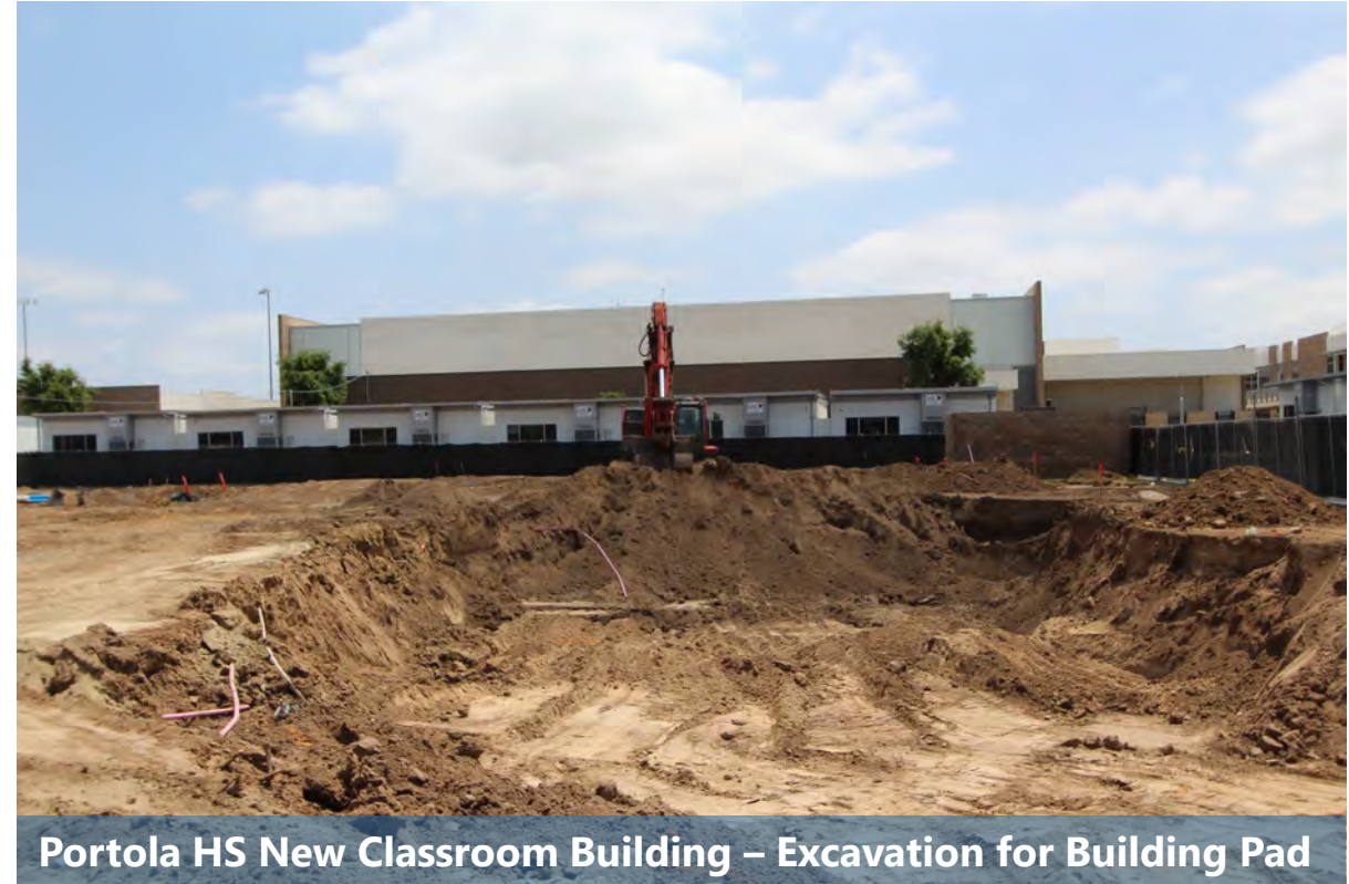
Portola HS New Classroom Building – Excavation for Building Pad
