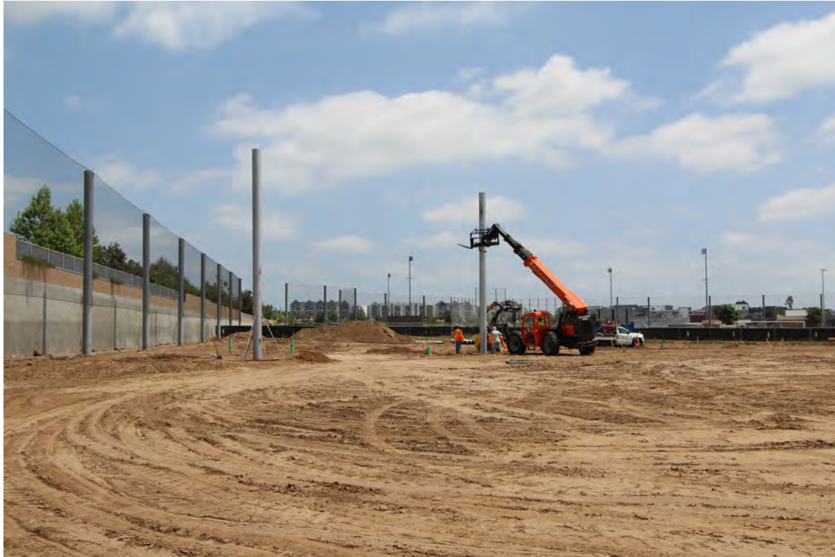
Portola HS Field Renovation – Installing Poles for Netting
