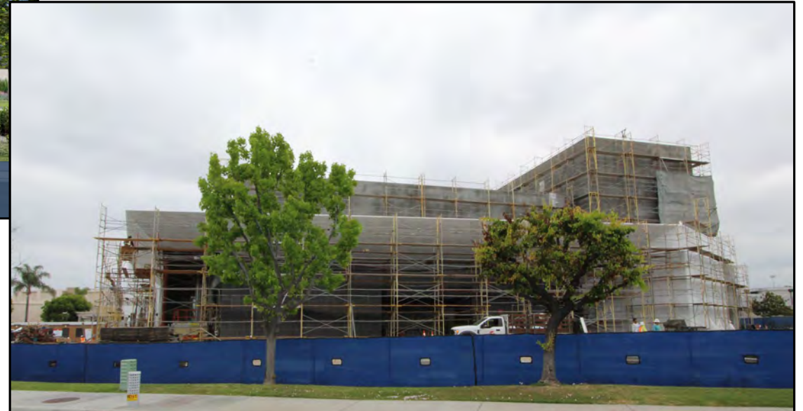
Street View (Walnut Avenue) - Under Construction
