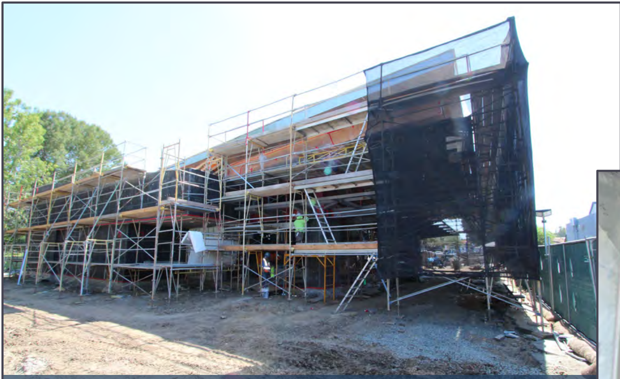
Plaster at exterior of MPR Building
