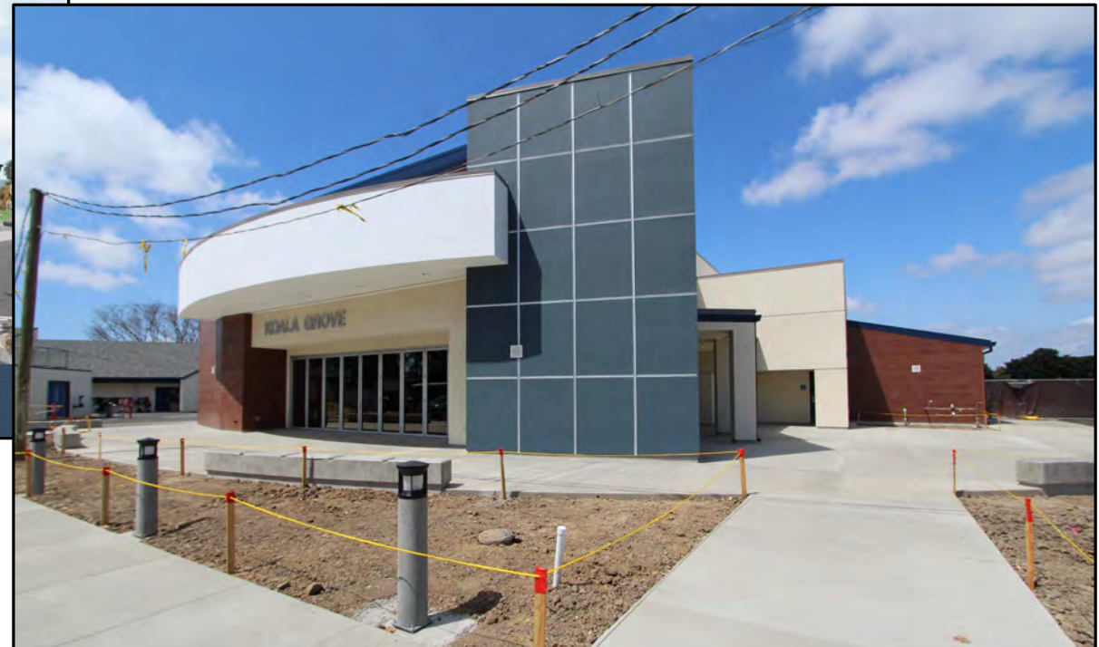
Exterior of new MPR Building - Under construction
