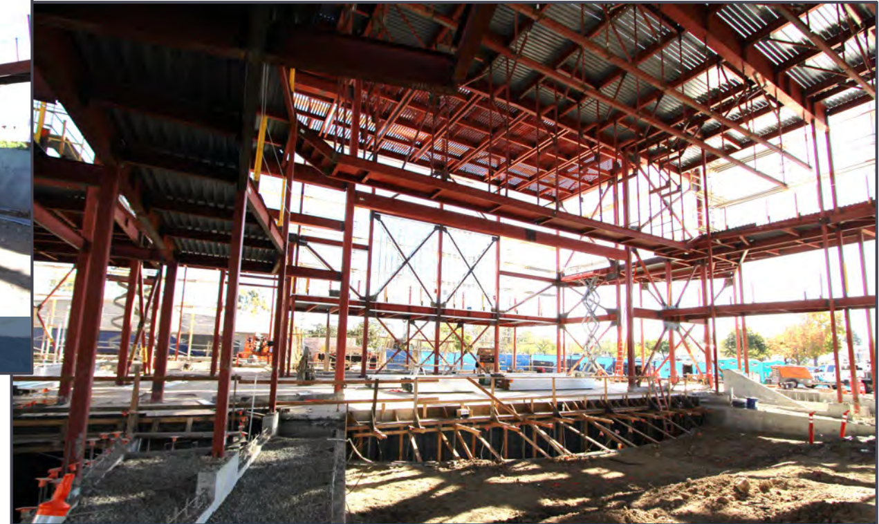
Grading at house floor (looking towards stage)
