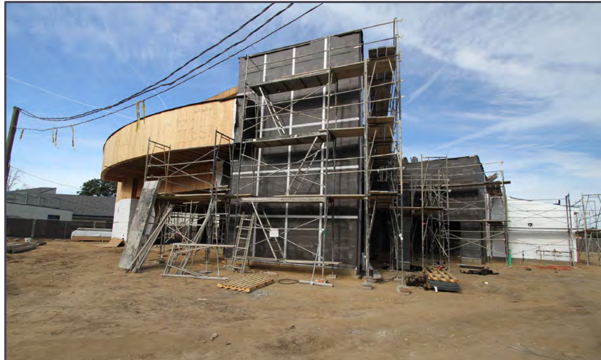
Exterior of new MPR Building – Scaffolding for plaster system
