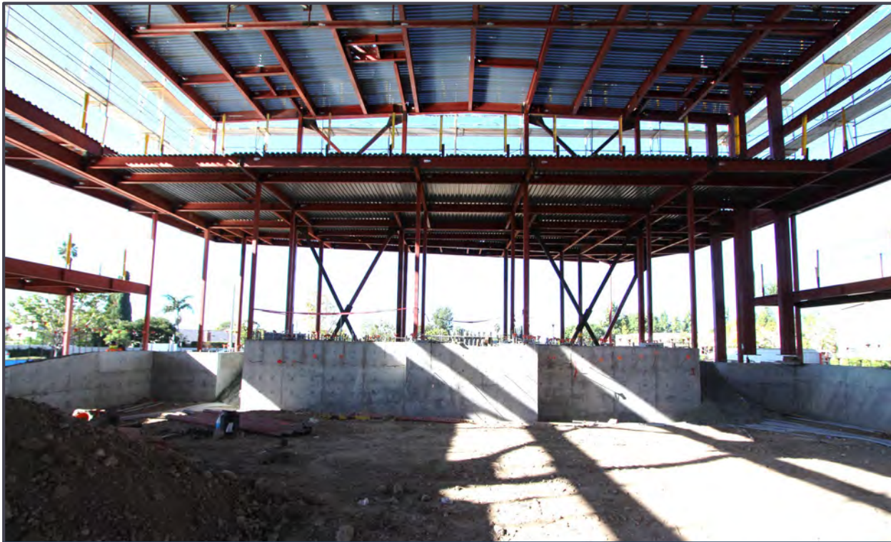
Grading at house floor (looking towards house seating)
