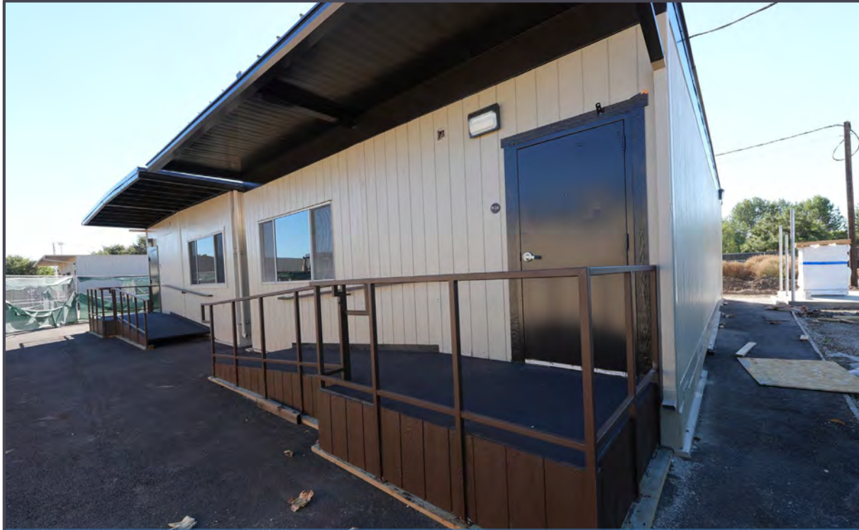
Adult Education Relocatable Classrooms - Exterior
