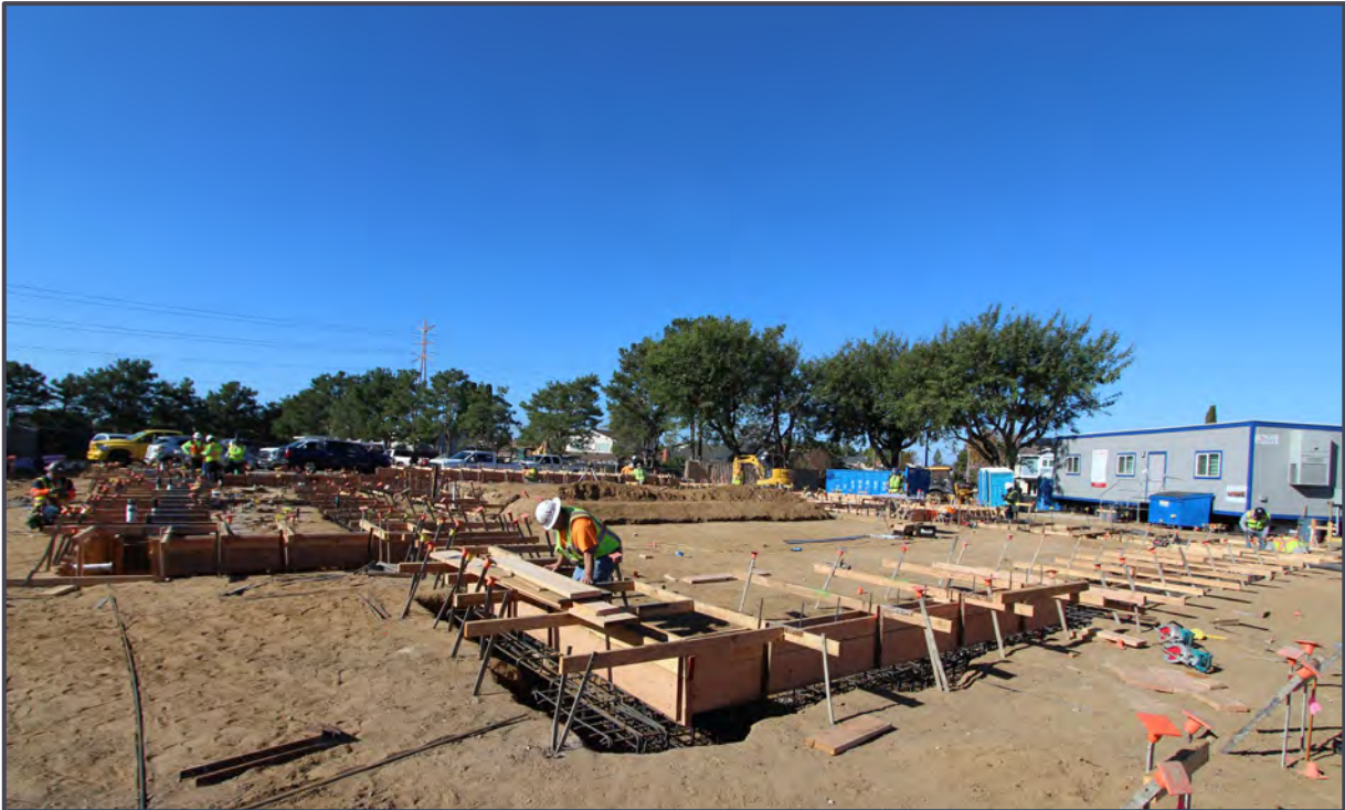
Stem wall formwork at front of MPR Building
