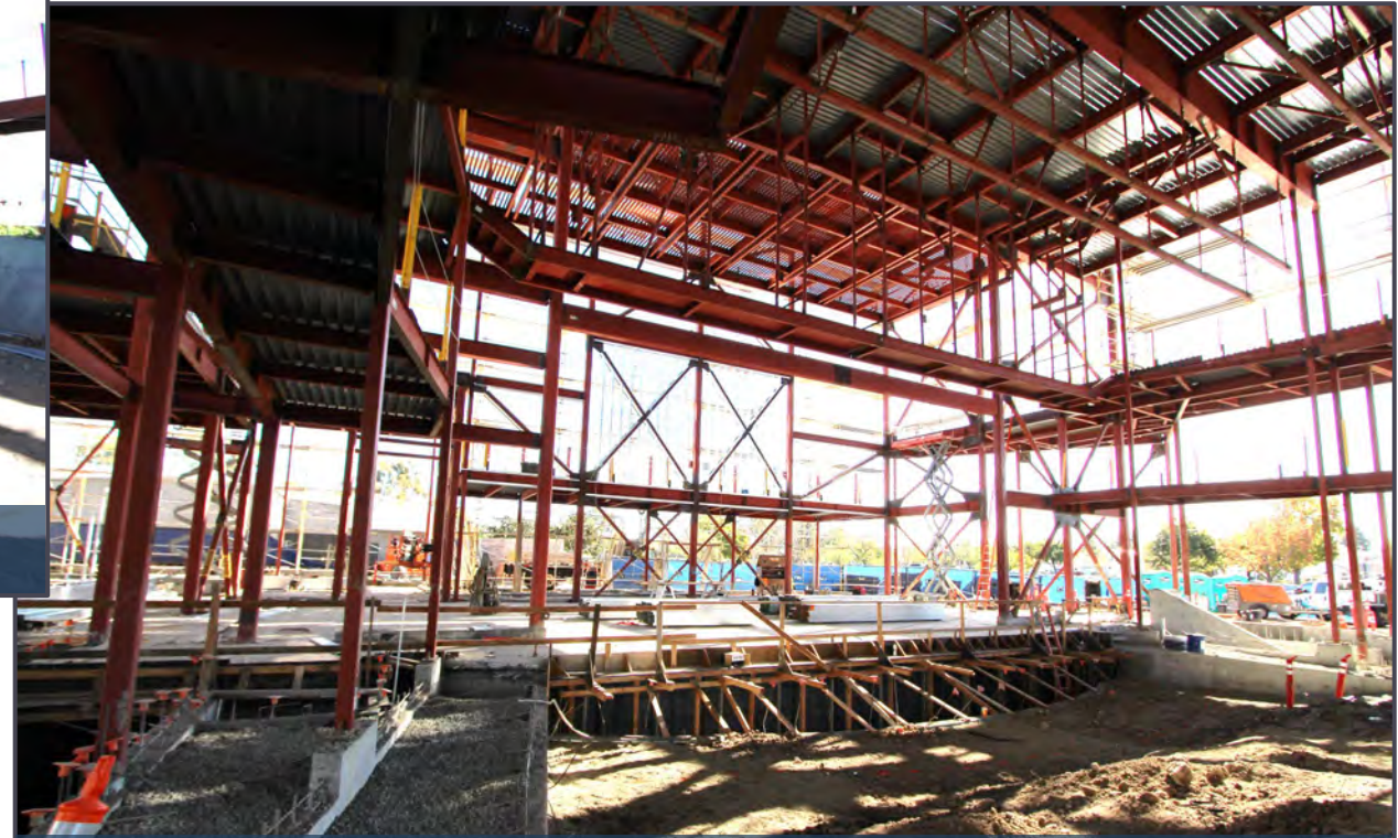
Grading at house floor (looking towards stage)
