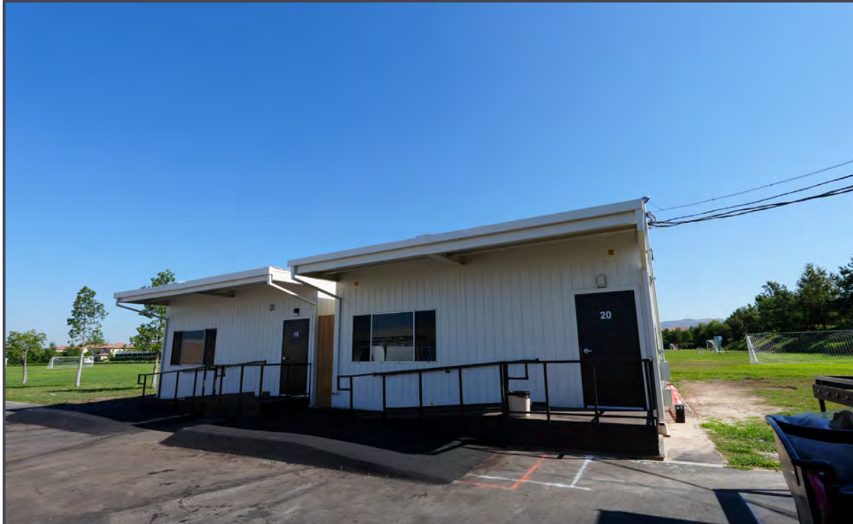
Relocatable Classrooms – Exterior
