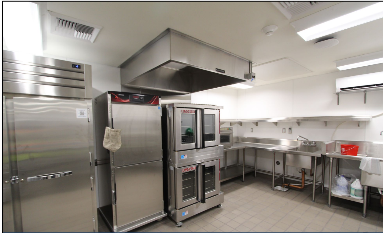
Nutrition Service renovation/expansion – Completed
