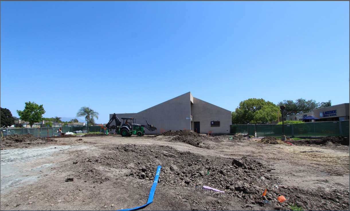
New Music Classroom – Site Demolition
