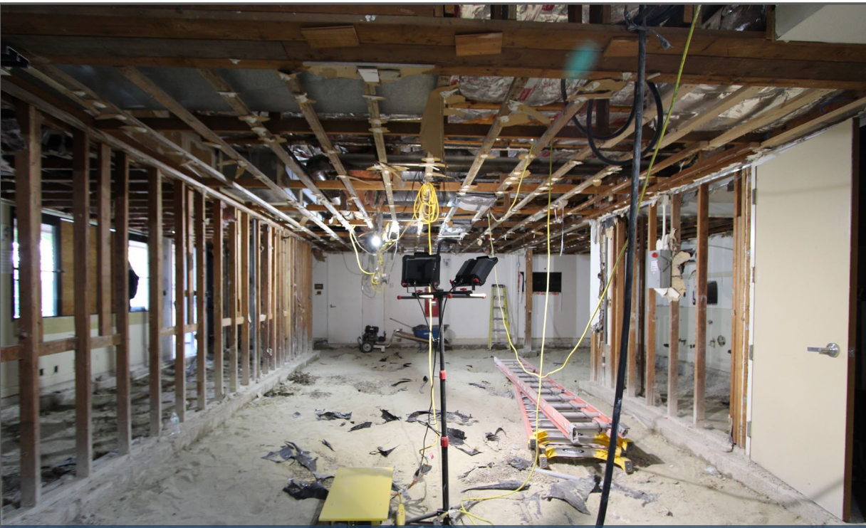
Nutrition Services – Demolition of Speedline Area
