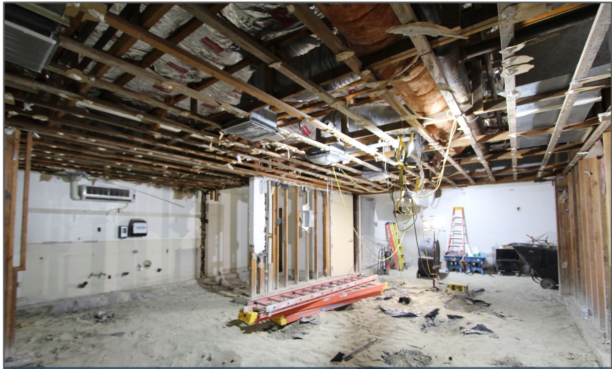
Nutrition Services – Demolition of Speedline Area
