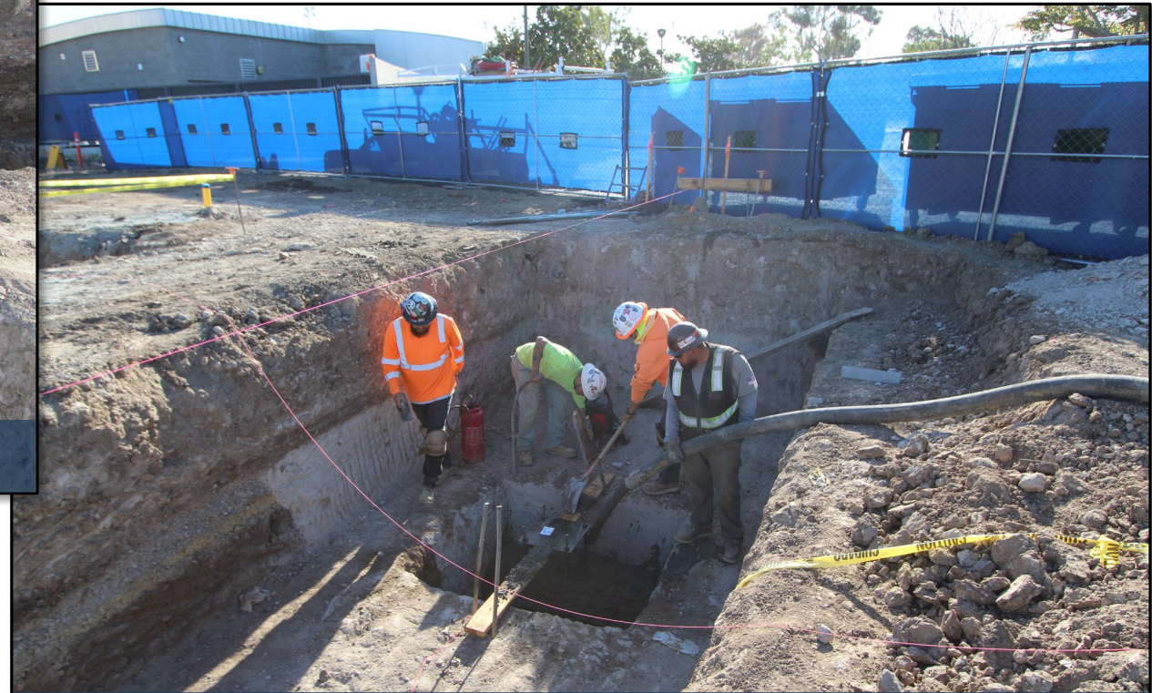
Increment No. 1: Building footings
