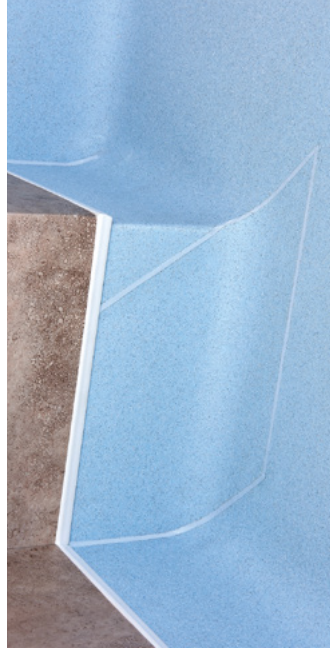
Figure 3.9 External corners 'wrap around method'
