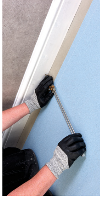
Figure 3.2 Scribing the wall profile
