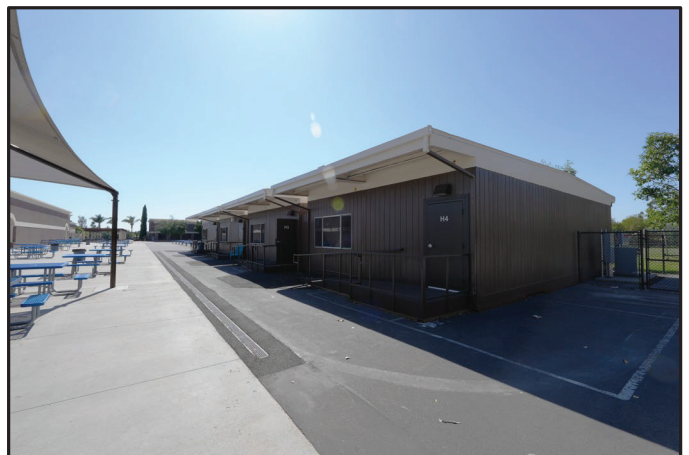
Jeffrey Trail Middle School Relocatable Classroom Buildings
