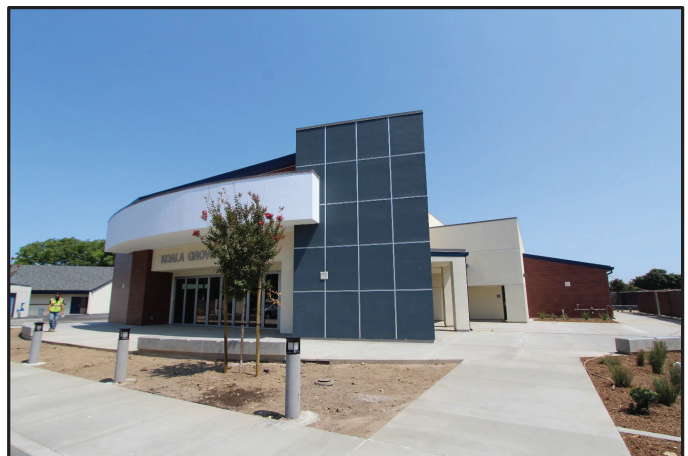
Measure E Culverdale Elementary School New Multipurpose Building
