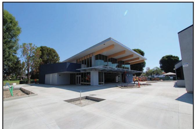
Measure E Santiago Hills Elementary School New Multipurpose Building
