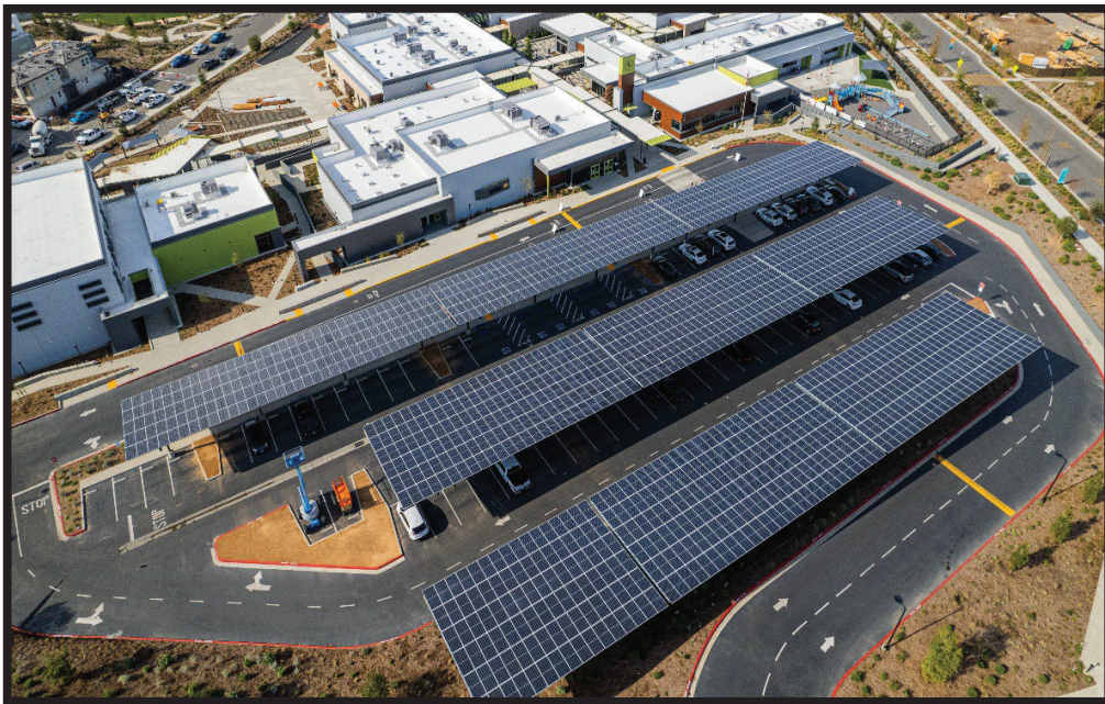
Solis Park School Solar Vehicle Shade Structure
