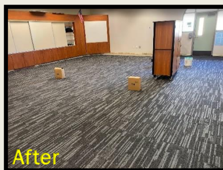
Woodbury Elementary Flooring Replacement
