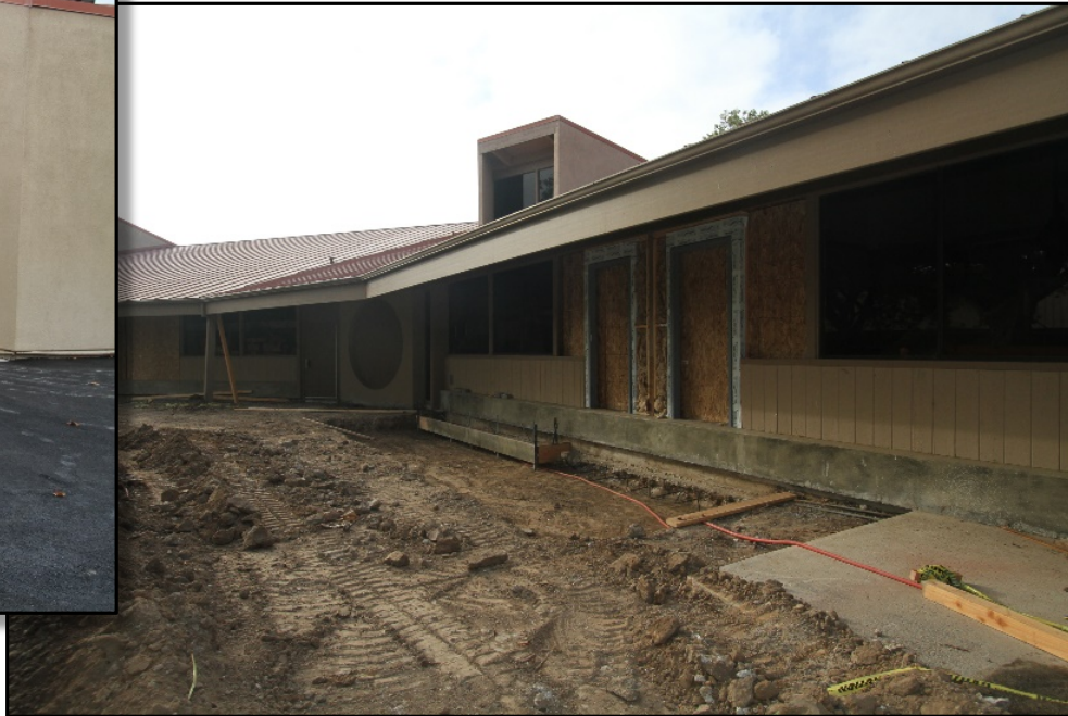
Picture 4: New door frames. Accessible improvements at doorways.
