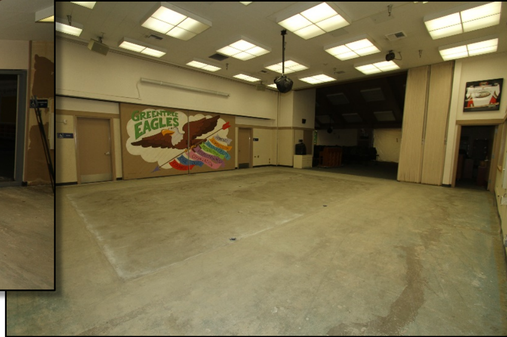
Picture 4: Concrete in-fill at multipurpose room.
