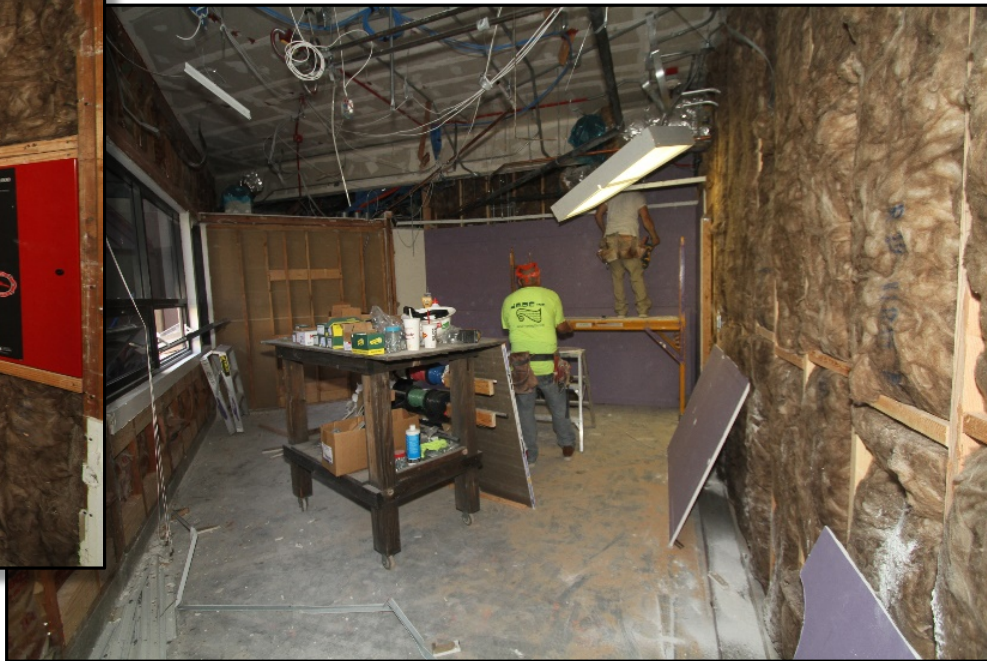
Picture 2: Wall installation and drywall in teacher workroom.
