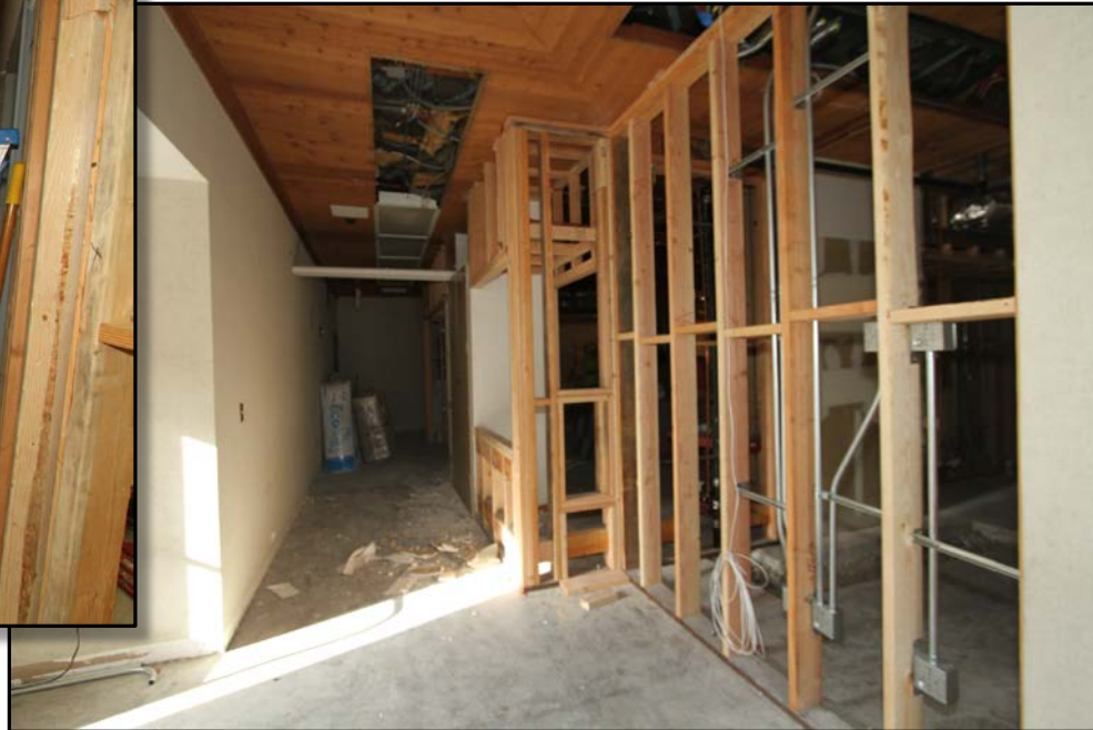
Picture 4: New student commons. Wood framing, and electrical rough-in.
