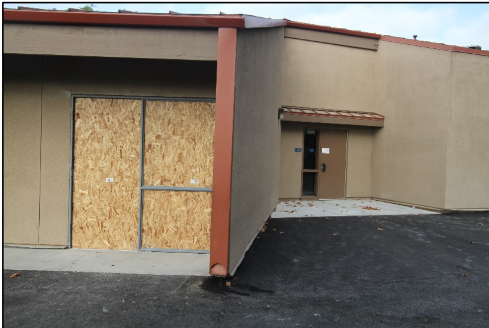
Picture 3: New door frames and sidelites at classrooms. New concrete pads and asphalt to improve drainage.
