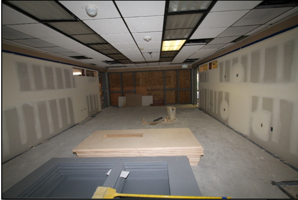
Picture 1: New student commons. Drywall and tape on walls. New storefront door opening. New doors in foreground.
