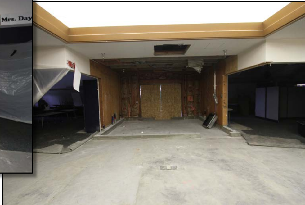
Picture 2: New accessible student restrooms. Concrete curbs for new walls. Classroom openings ready for new door frames.
