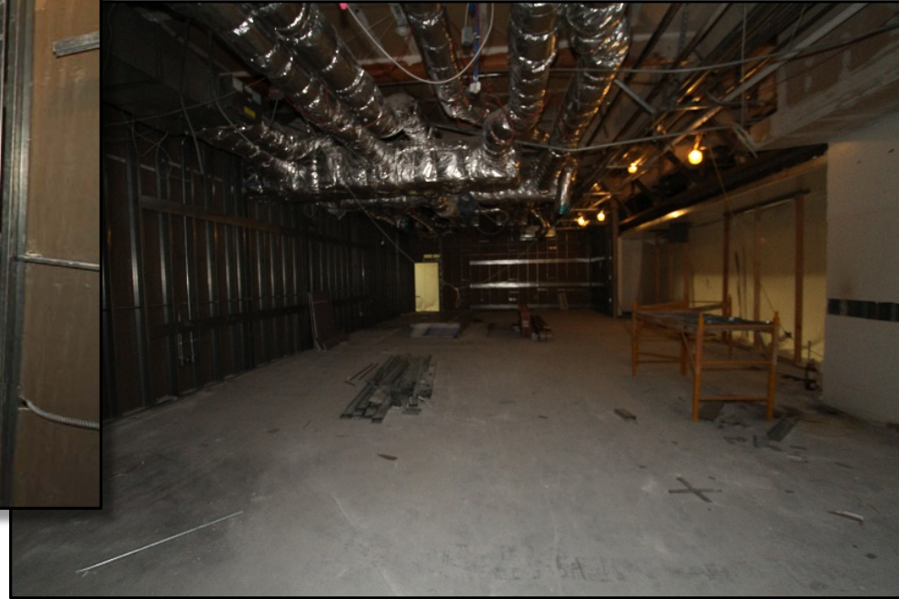
Picture 2: New music classroom. Metal stud framing, new ductwork, and opening to multipurpose room stage.
