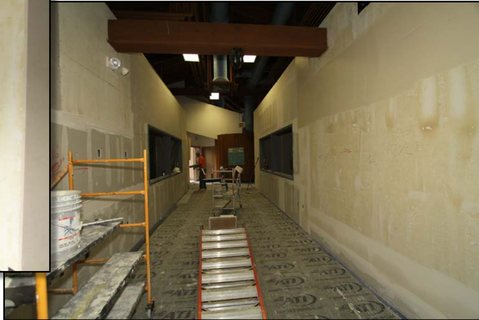
Picture 2: New student commons. Drywall and tape on walls.
