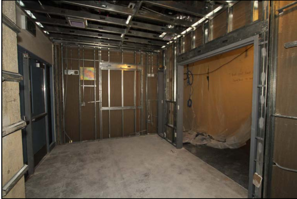
Picture 1: New entrance into administration area. Metal stud framing and new door opening.
