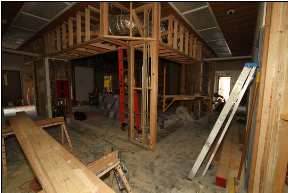
Picture 3: New student commons. Wood framing, electrical rough-in, and mechanical ductwork.
