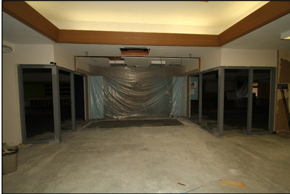
Picture 3: Installation of new door frames and sidelites.
