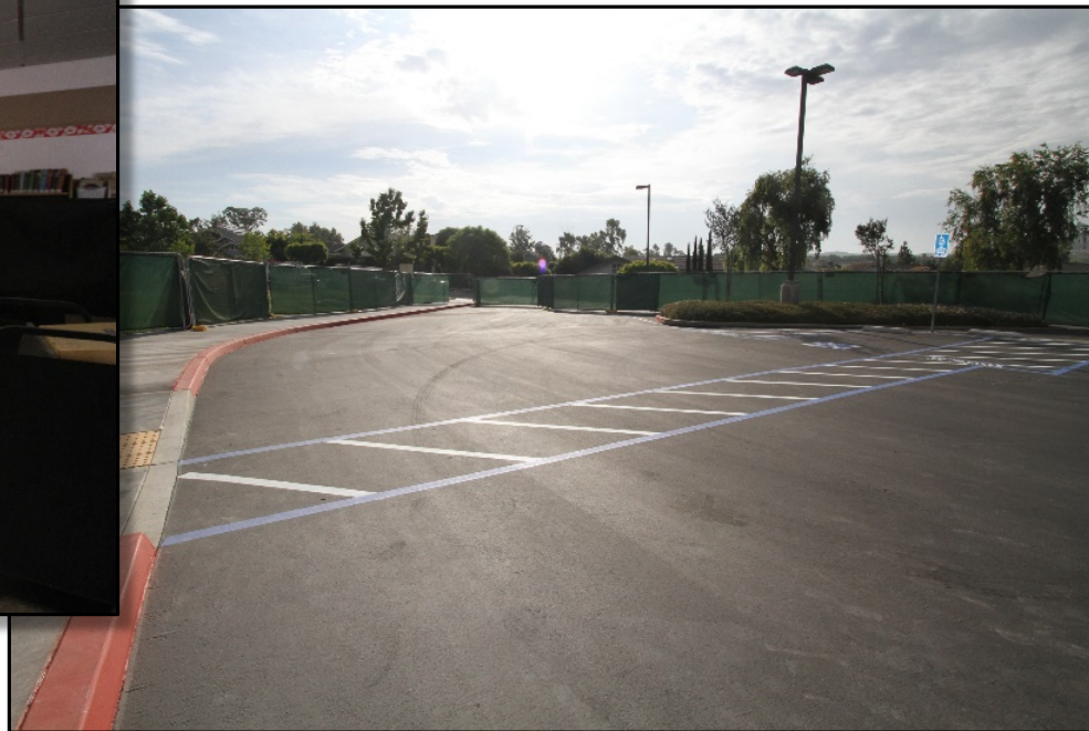
Picture 4: New accessible ramp. New curb, gutter, and walkway to street. New asphalt slurry and striping.
