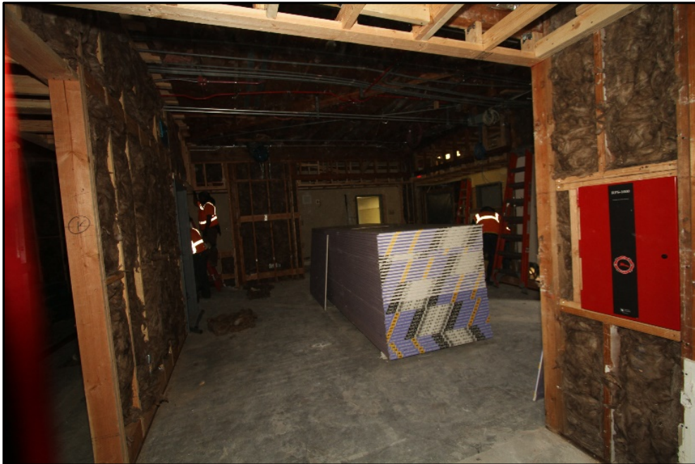
Picture 1: Wood framing and wall insulation in new student commons.
