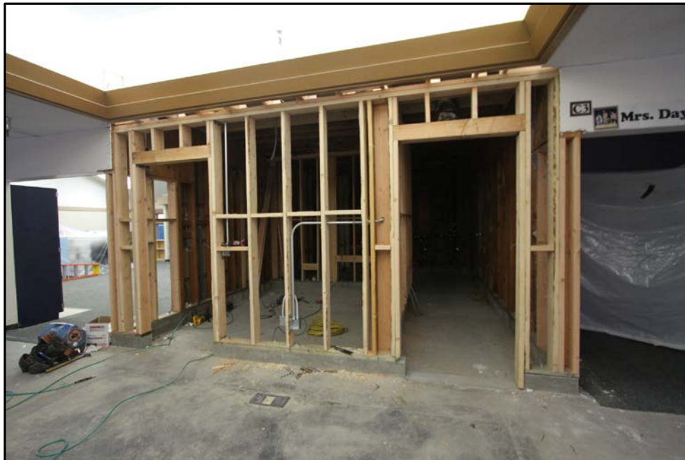
Picture 1: New accessible student restrooms. Wood framing and electrical rough-in.
